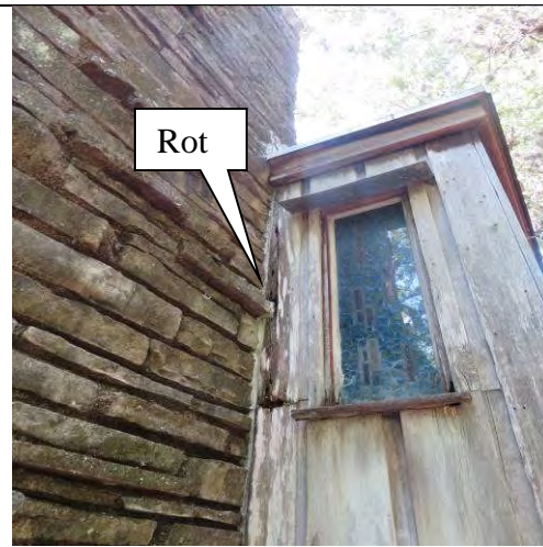
16. Wall rot &amp; leak at "chimney" addition
