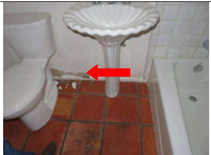
68. Water damage at bathroom ext'r wall
