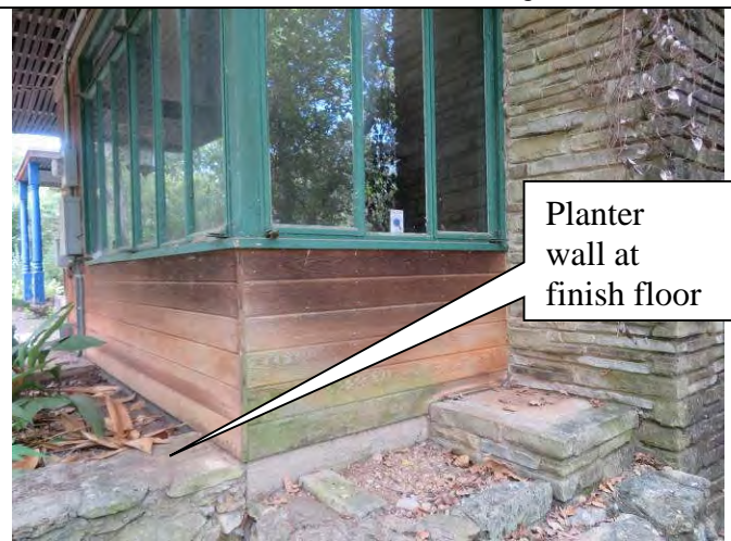
20. Deteriorated siding
