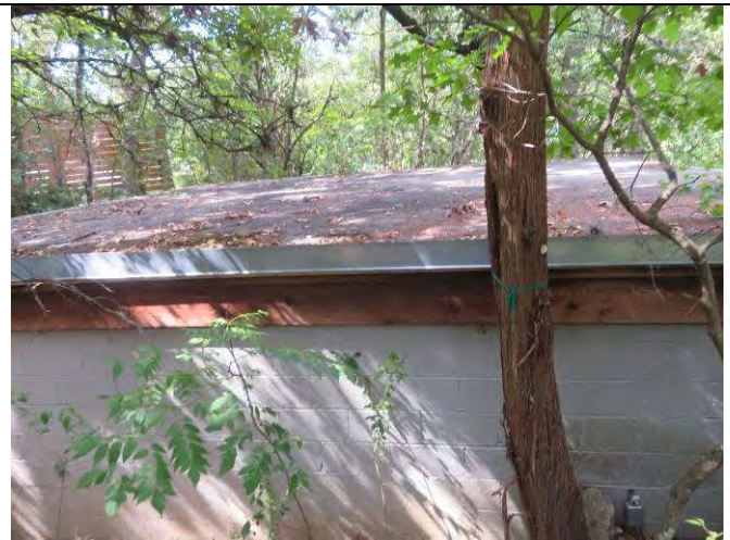
6. Garage roof ponds water
