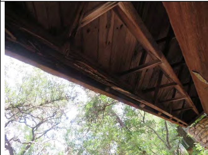
5. Rot under garage roof overhang
