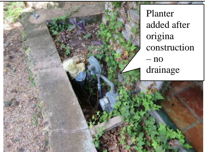
12. Gas meter at original grade
