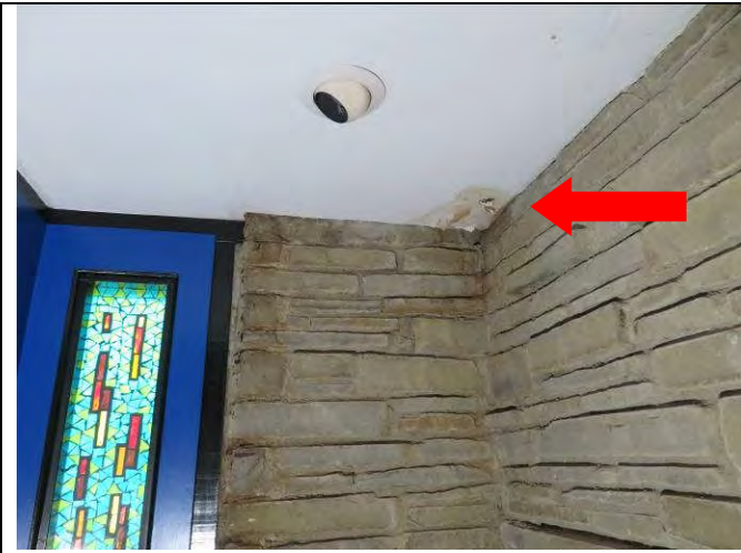
69. Water leak at room next to chimney
