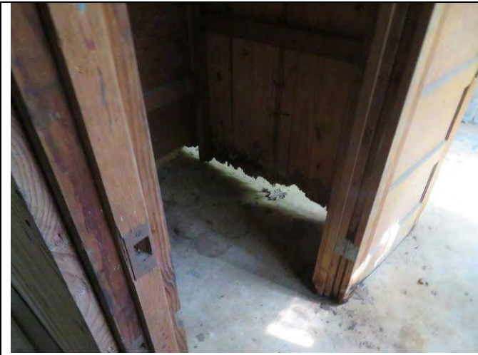
9. Rotted garage walls - typical
