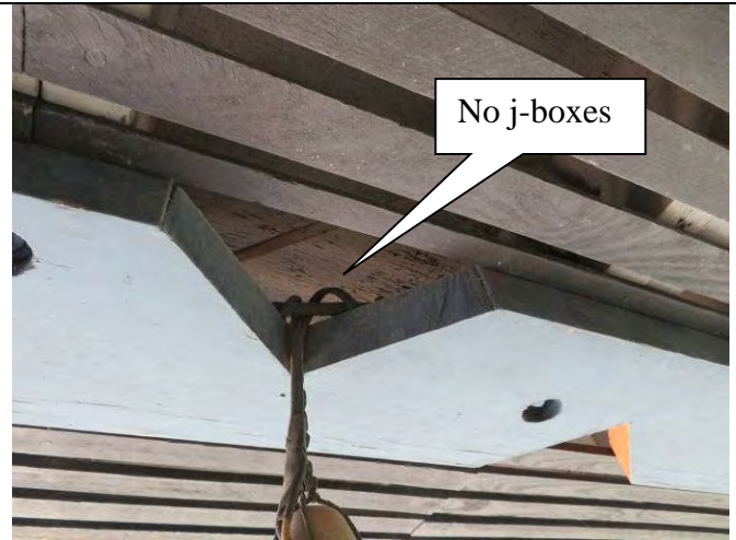
48. Improper wiring methods and materials
