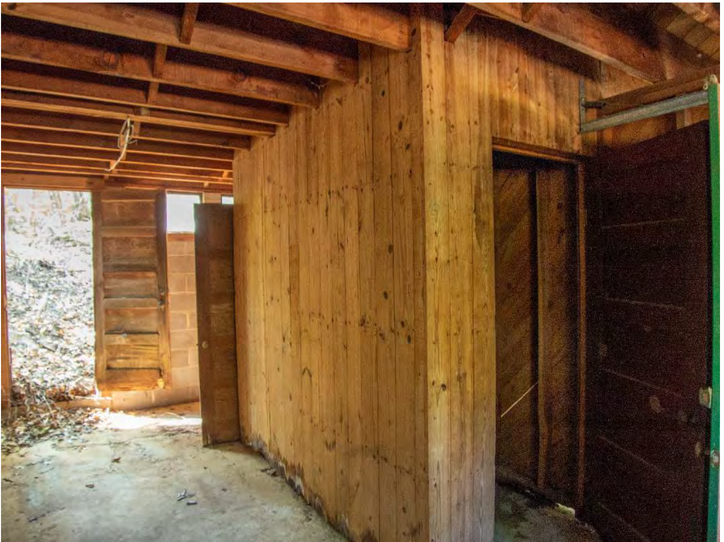
Figure 24. Interior of garage exhibits extensive rot resulting from site grading and drainage challenges
