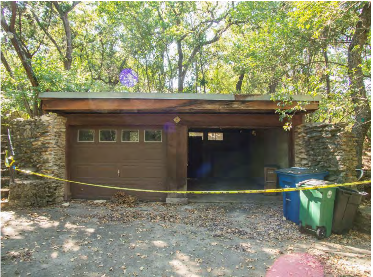
Figure 23. Garage has rotten fascia
