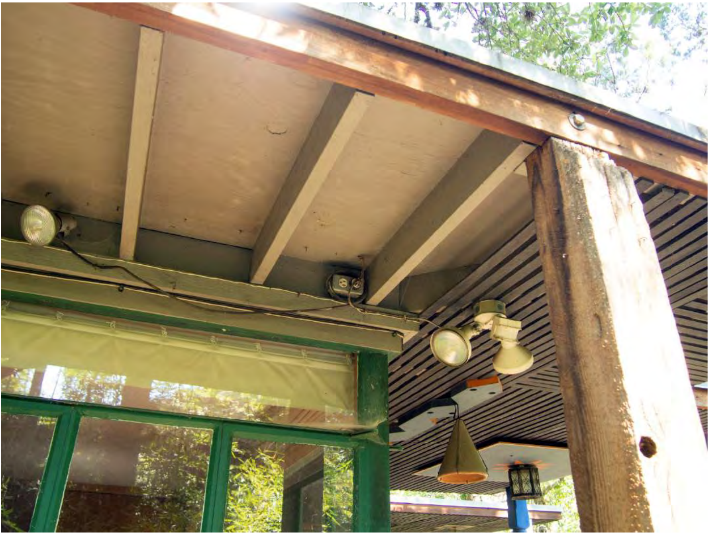
Figure 22. Retrofitted lighting is not hardwired and does not meet code
