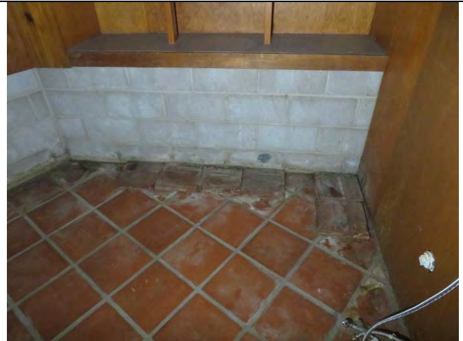
66. Water leaks at exterior wall - utility
