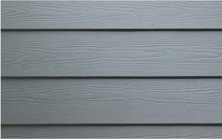
EXISTING SIDING: PTD WOOD SHIPLAP
