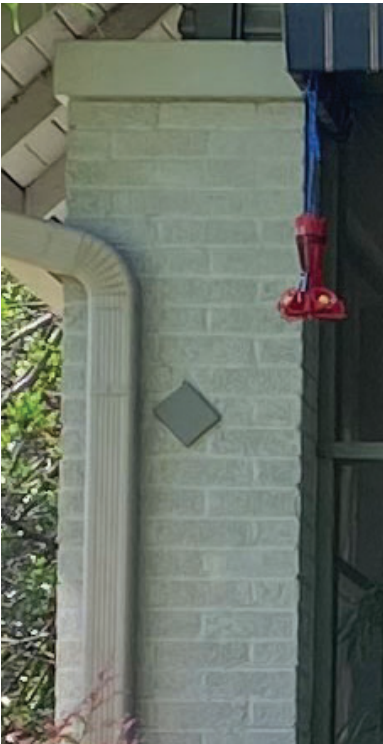
1. BRICK IS BEING USED TO CLAD PORTION OF ADDITION
