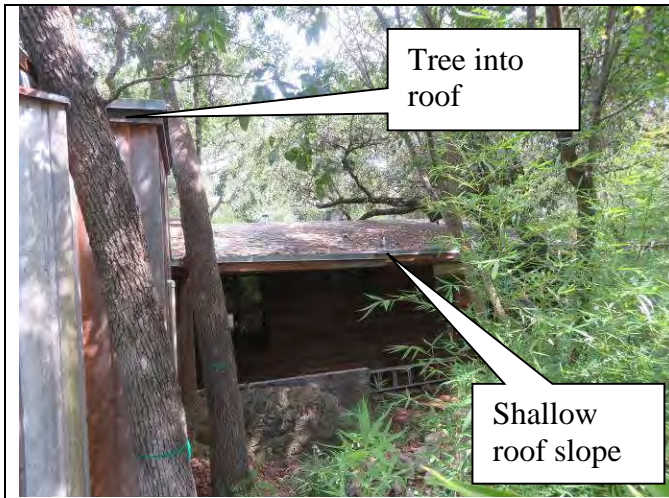
33. Shallow pitch roof at rear
