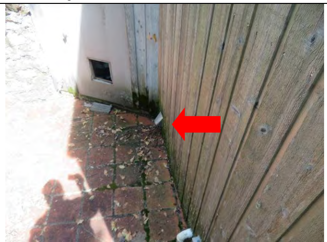
38. Rot / leaks at utility room wall base
