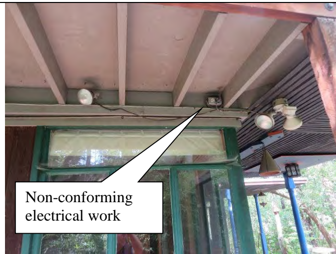
45. DIY electrical wiring and fixtures
