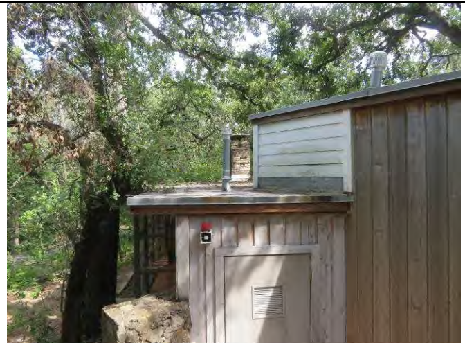
40. Roof flashing at flat roof
