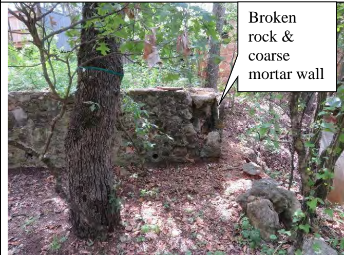
11. Typical stone rubble wall construction
