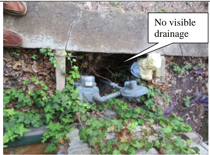
42. Gas meter pit (looking down)
