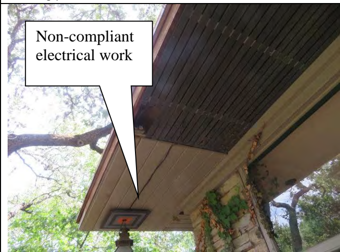
13. Varying soffit materials
