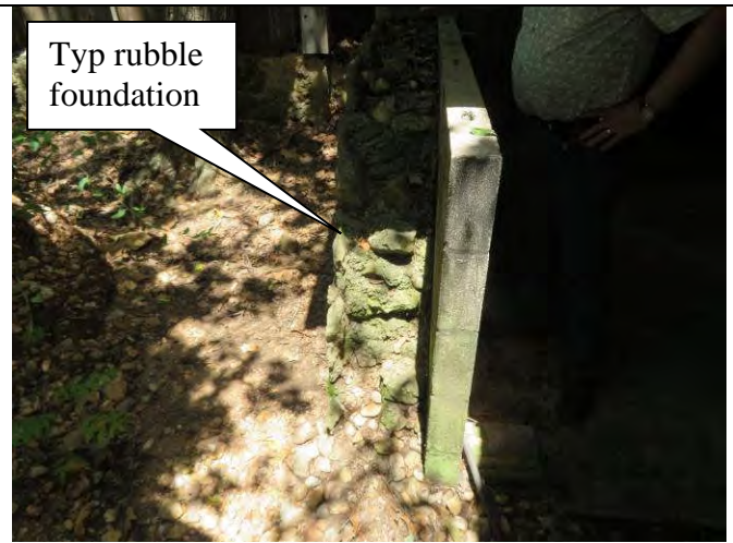
34. Typ rubble filled foundation wall
