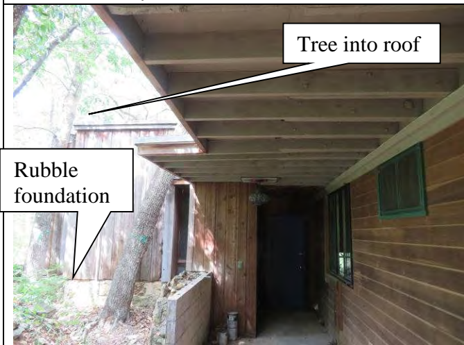
35. Roof sag at extended overhang
