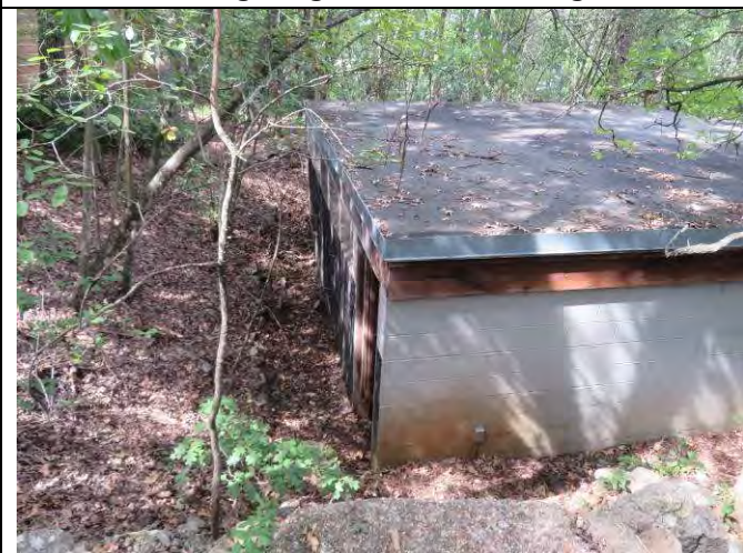
7. Soil above garage floor grade on 3 sides
