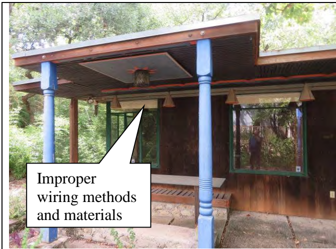
57. Light fixtures not rated for outdoor use
