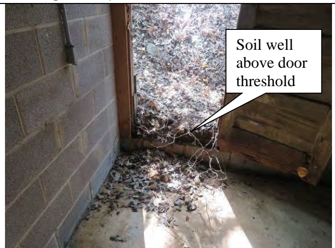
8. Soil above garage floor / water leaks
