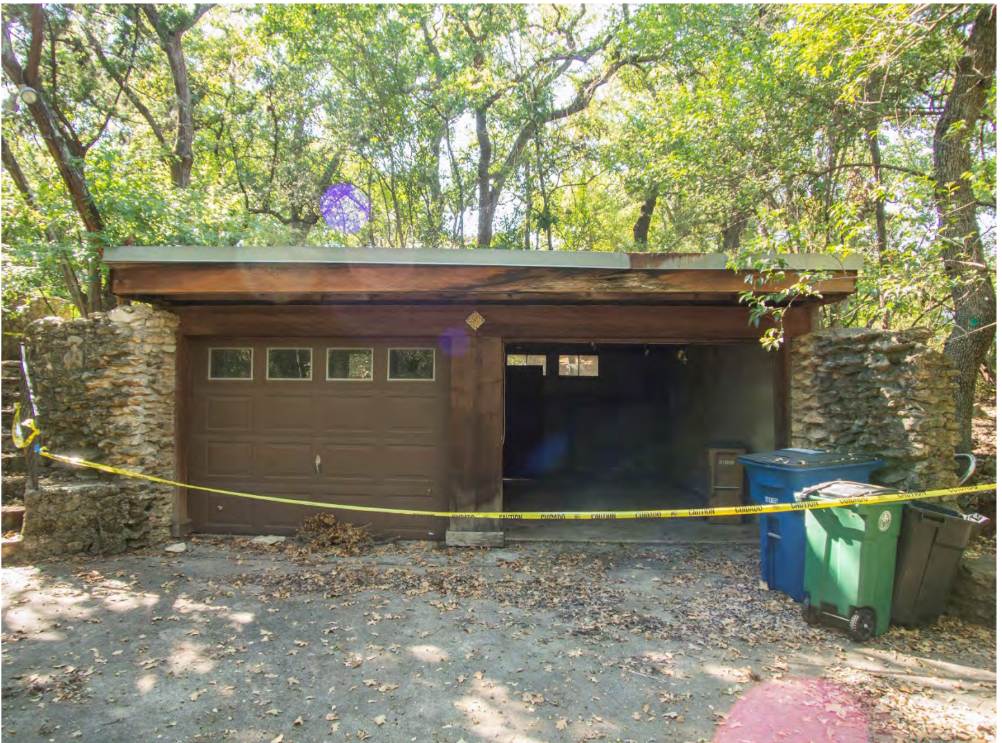
Figure 23. Garage has rotten fascia
