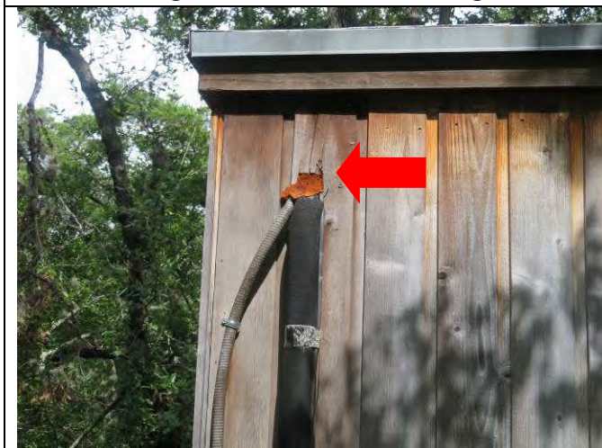
37. No flashing at wall penetration
