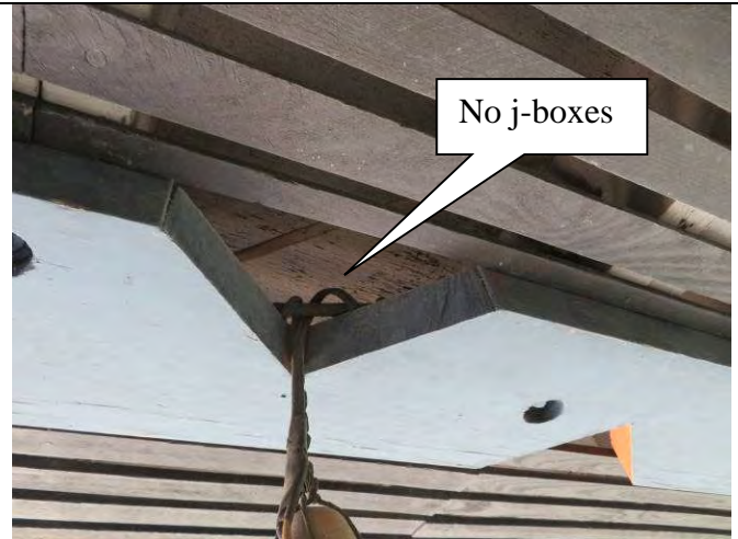
48. Improper wiring methods and materials
