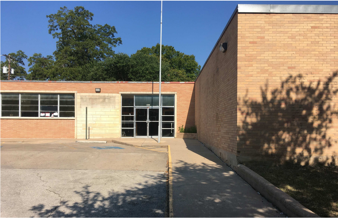
EAST DETAIL (STOREFRONT - 2 BRICK TYPES)
