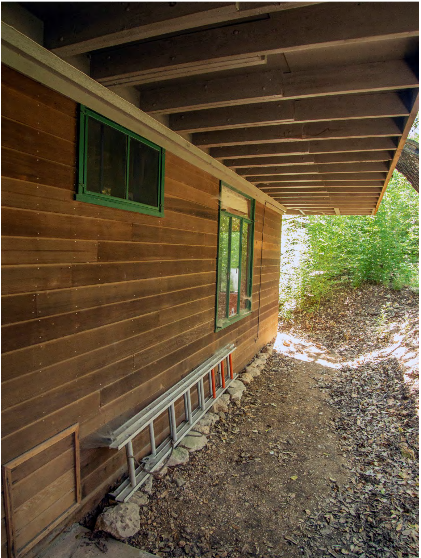
Figure 17. Extended roof overhang
