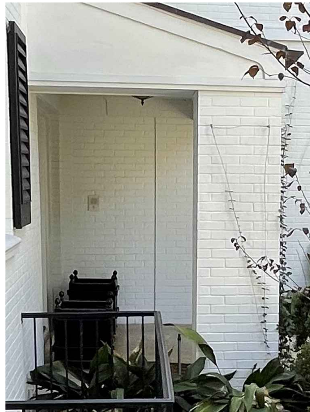
EXISTING PORCH CORNER NORTH ELEVATION Illustrates: Existing decorative brick header. Above brick infill (brick infill to be demolished a replaced with a steel door painted to match existing window color to show it is new in material but blend in with color.) re: Cad Exterior elevations and Historical plan for historic opening locations.
