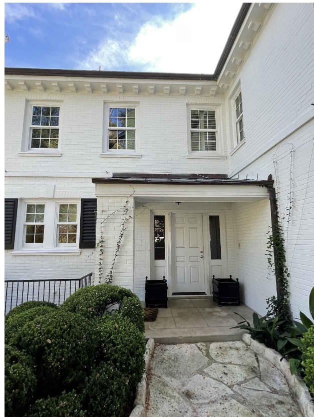
EXISTING PORCH FRONT ELEVATION ON REAR-EAST ELEVATION Illustrates: Opening under existing brick decorative header. New window to sit within this opening. Remaining area will be unfilled with brick, but a minor delineation will be left to illustrate infill.
