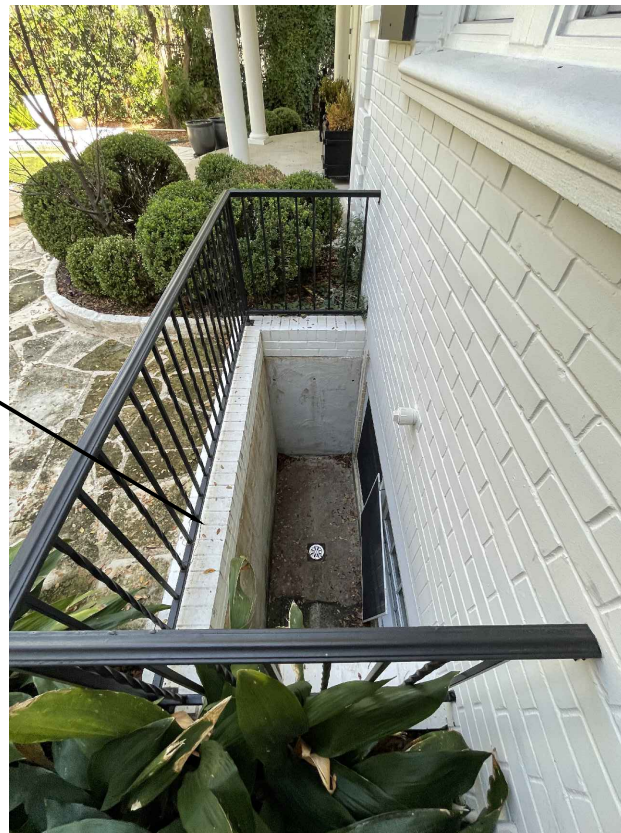
WINDOW WELL DETAIL IMAGE Illustrates: brick at window well NOT HISTORIC per window well detail on this sheet.
