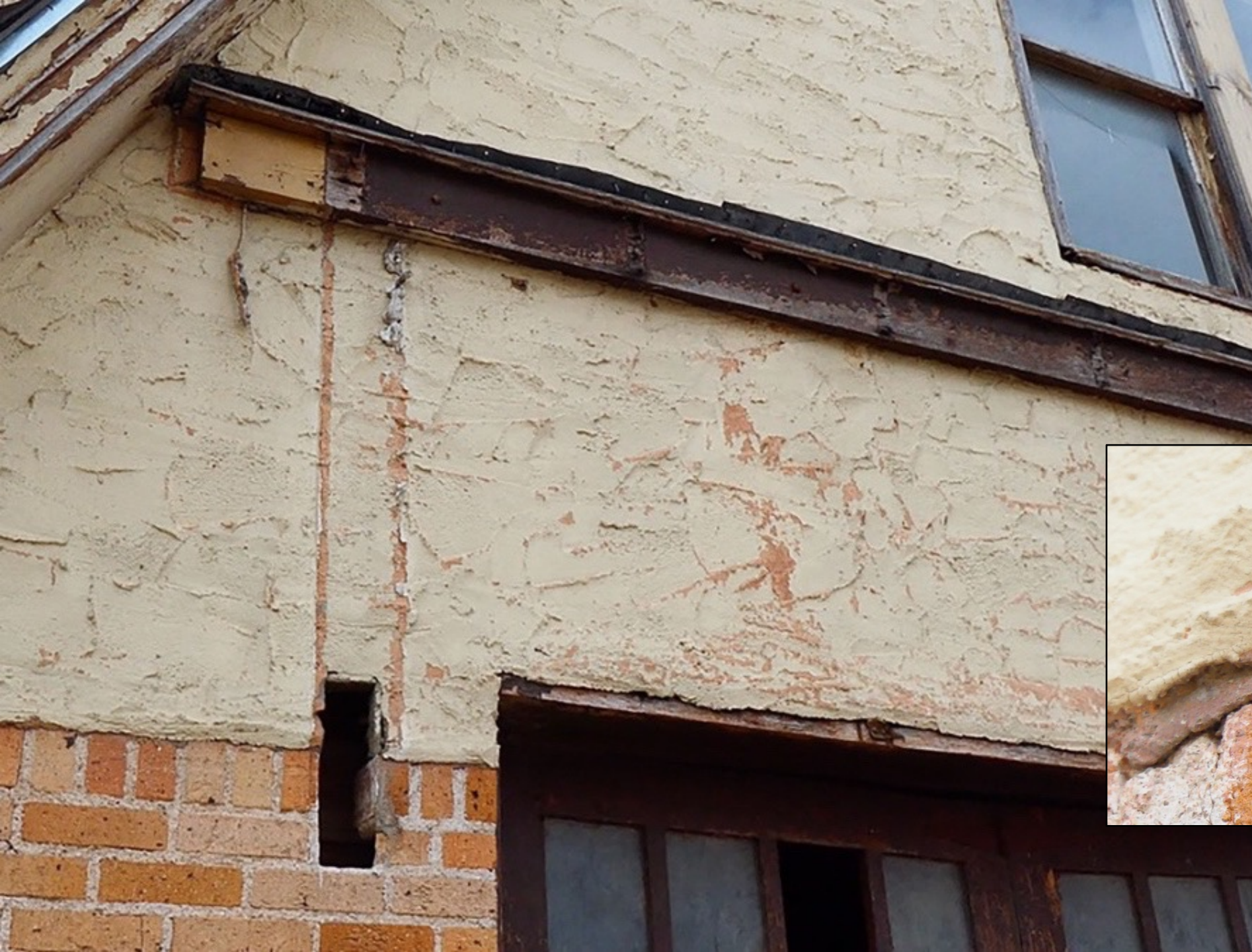
Garage – Stucco and evidence of original awning
