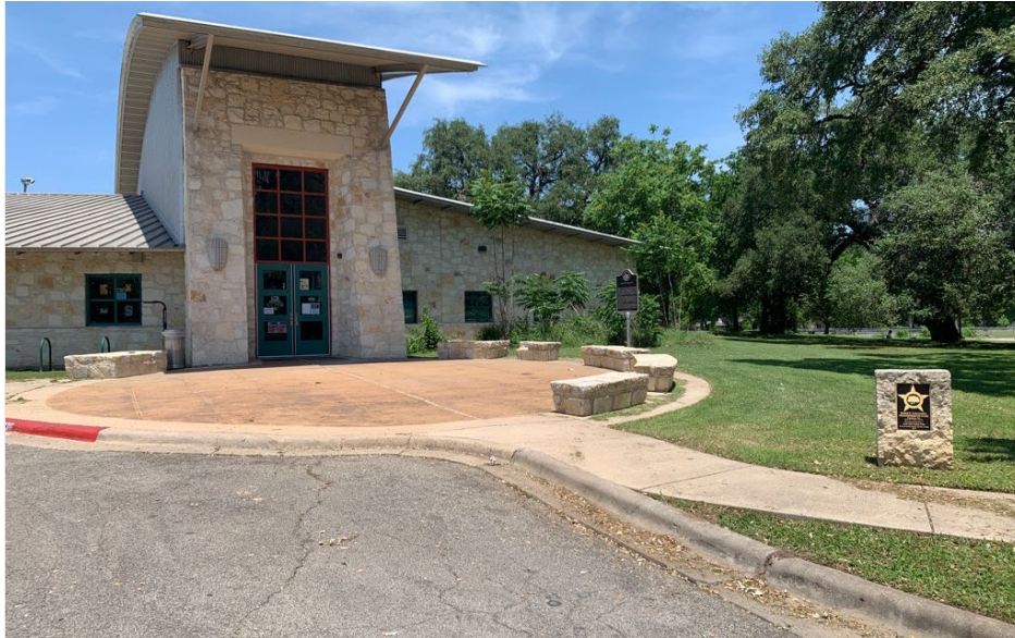
Conditions at Parque Zaragoza before rehabilitation began
