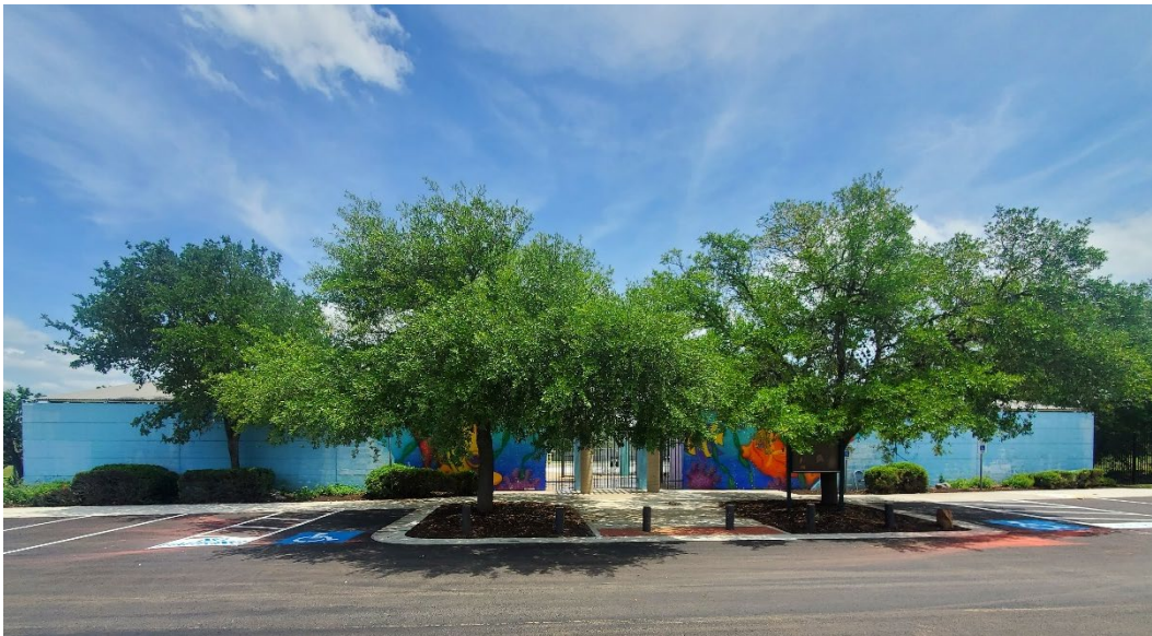
Parking lot improvements at Dick Nichols District Park
