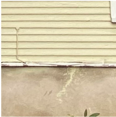
2. STUCCO IS BEING USED FOR LOWER PORTION OF ADDITION
