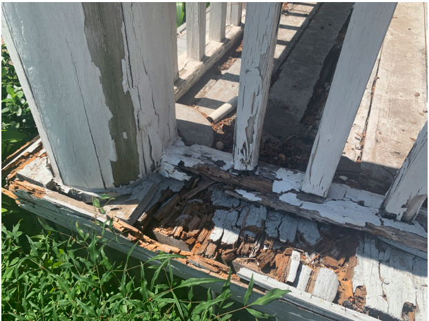
REPAIR DAMAGED PORCH DECK AND REPLACE RAILING
