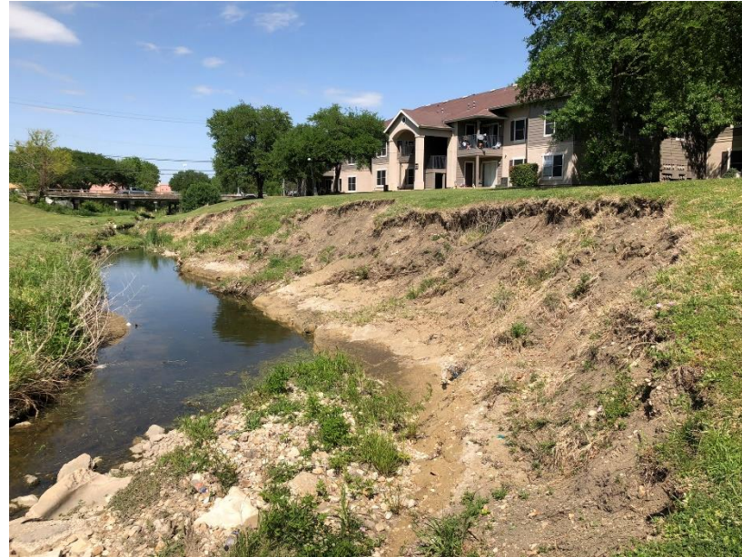
Erosion along Country Club Creek West, looking north towards E Riverside Dr
