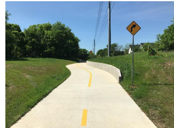
Burleson Rd to Ventura Dr Off-street trail in Austin Energy easement
