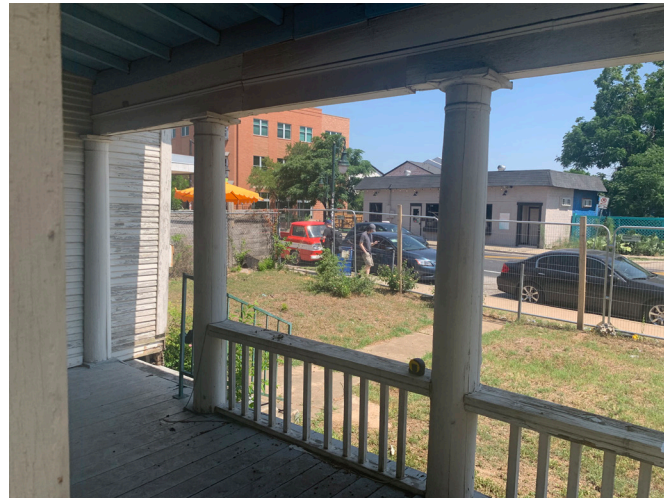
NON-ORIGINAL ALTERATIONS AT DEEPER COVERED PORCH ROOF SUPPORT BEAMS, SHORTENED COLUMNS AND PLYWOOD AT COVERED PORCH CEILING.
