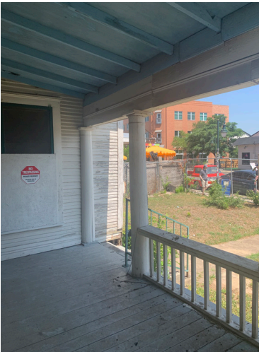
NON-ORIGINAL ALTERATIONS AT DEEPER COVERED PORCH ROOF SUPPORT BEAMS, SHORTENED COLUMNS AND PLYWOOD AT COVERED PORCH CEILING.
