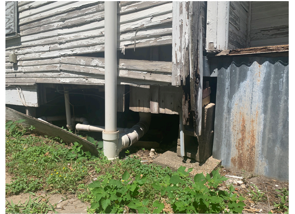
DETERIORATING FOUNDATION, METAL SKIRT AT PORCH DECK AND EXPOSED SOIL STACK.
