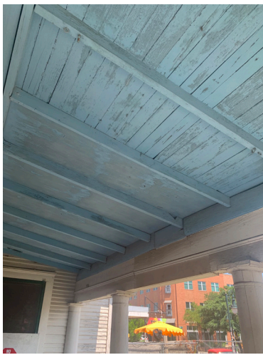
NON-ORIGINAL ALTERATIONS AT DEEPER COVERED PORCH ROOF SUPPORT BEAMS, SHORTENED COLUMNS AND PLYWOOD AT COVERED PORCH CEILING.
