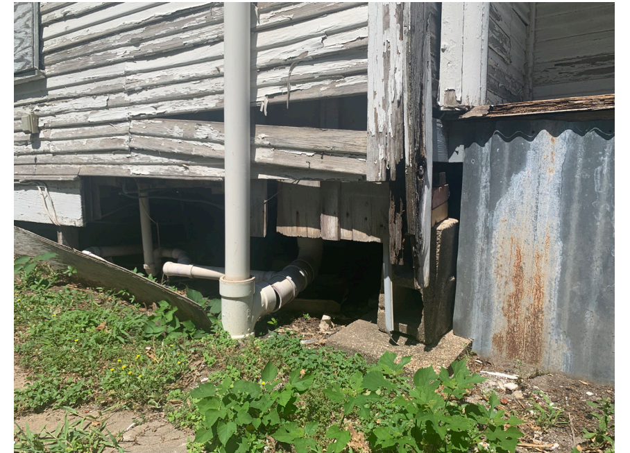
DETERIORATING FOUNDATION, METAL SKIRT AT PORCH DECK AND EXPOSED SOIL STACK.
