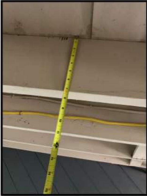
Figure 2: 2x8 floor framing at 16".
