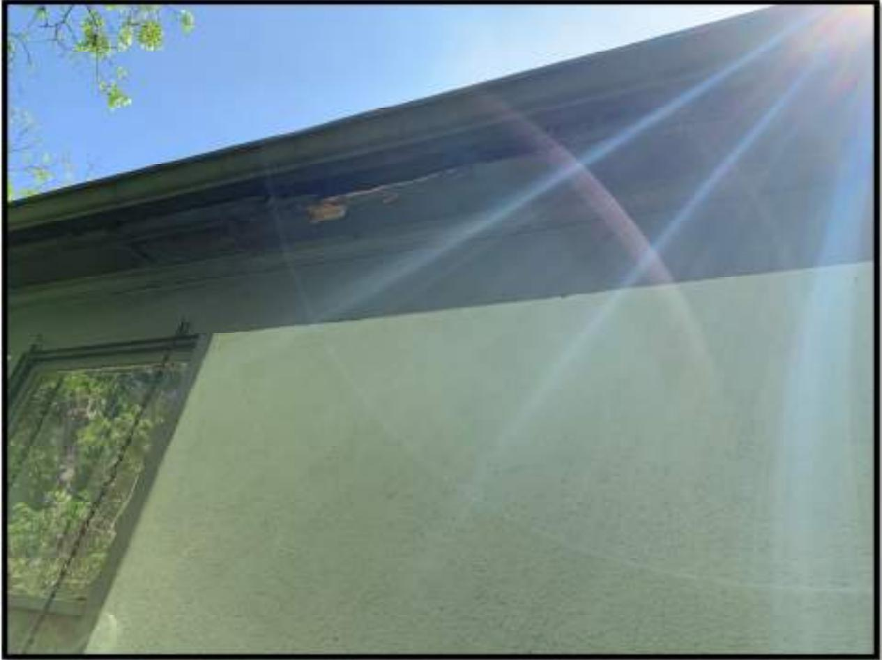
Figure 5: Rotted soffit on West side of ADU.
