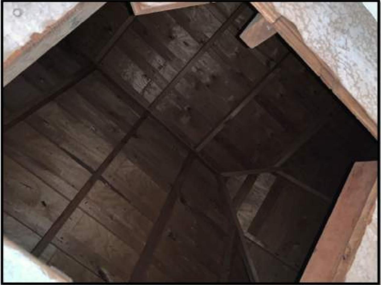
Figure 1: 2x4 roof framing at 24", 2x4 ridge beam, and 2x4 hip beam, note lack of vertical support at hip to ridge connection.
