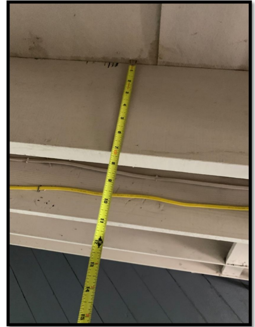
Figure 2: 2x8 floor framing at 16".
