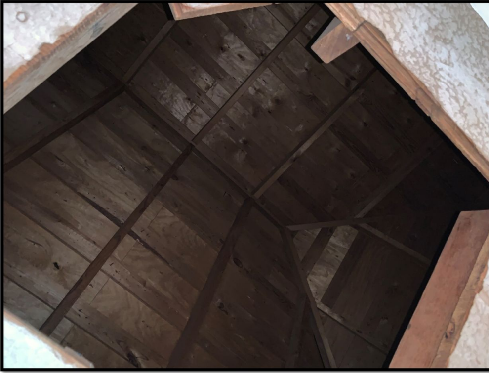
Figure 1: 2x4 roof framing at 24", 2x4 ridge beam, and 2x4 hip beam, note lack of vertical support at hip to ridge connection.
