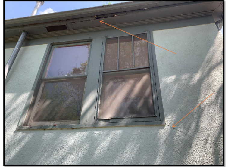
Figure 4: Rotting soffit and crack stucco veneer on rear wall
