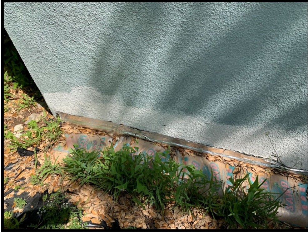
Figure 3: Rear wall, SW corner, sand bags, and soil built up above bottom plate.
