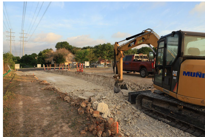
An excavator grades the ground to create a smooth and level base for the new trail (left). A surveyor measures the land slope (right).
