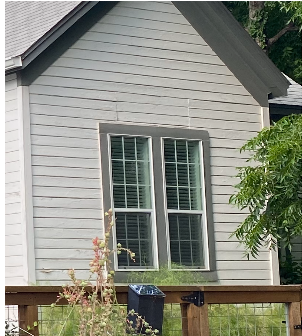
DETAIL SHOWING PATCHED SIDING / NON ORIGINAL WINDOWS AT 1400 GARDEN ST.
