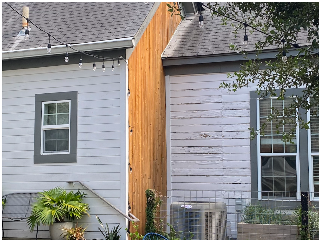
NEW VS. EXISTING ROTTEN SIDING AT 1400 GARDEN ST.
