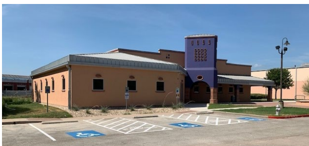
Cepeda Branch exterior
