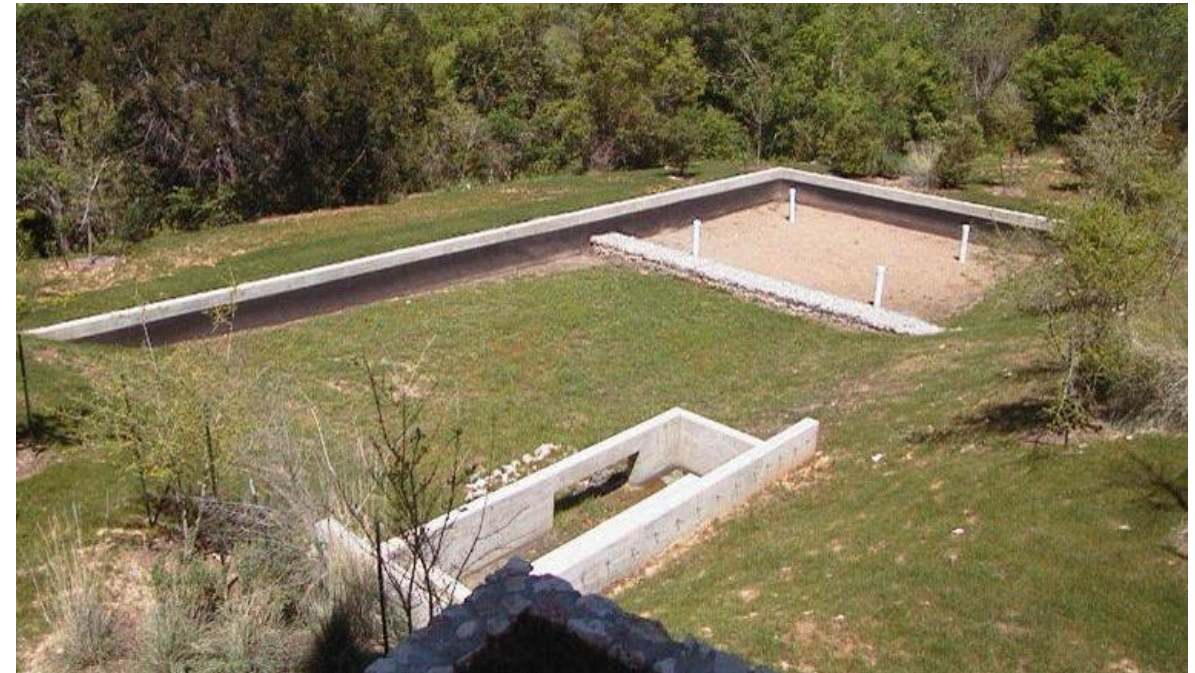
Conventional Stormwater Control (Sedimentation & Filtration Pond)
