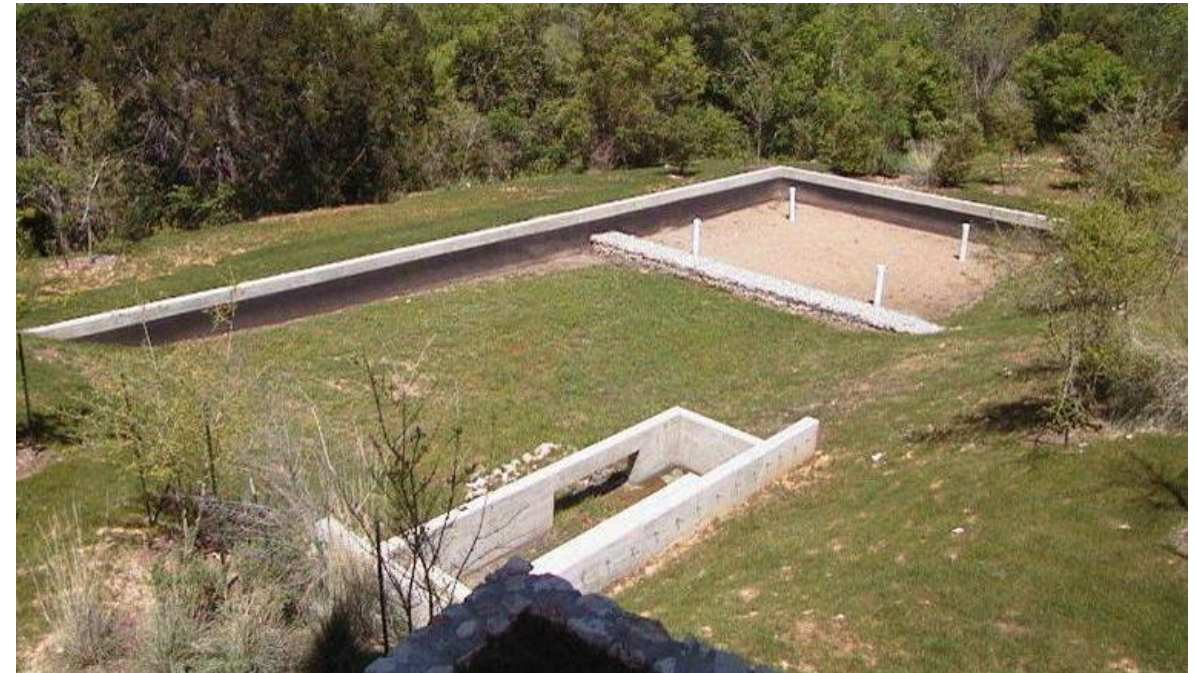
Conventional Stormwater Control (Sedimentation & Filtration Pond)
