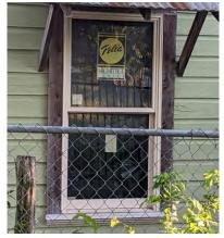
Clad-wood window Wood frame clad in aluminum frame; mimics the appearance of woodsash windows but with sharper manufactured edges.
