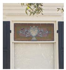
Leaded glass window A window composed of pieces of glass that are held in place with lead strips; the glass can be clear, colored, or stained.
