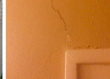
**Above left:** Parts of Austin have clay soils that move based on varying moisture conditions, and early slabs were not always properly reinforced. As a result, many historic slab-ongrade foundations have cracks as a result of settling.
