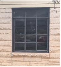
Steel-sash window Typically casement or fixed, with multiple lites.
