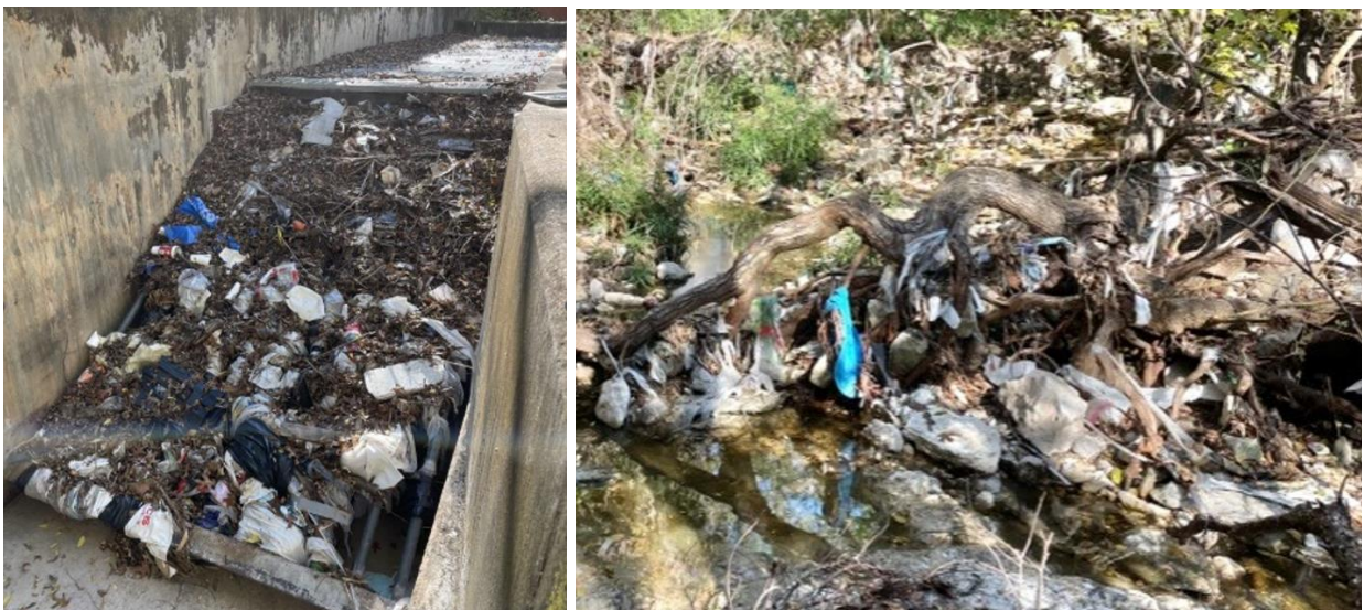
Figure 30. Trash detained by the rack (left) of the stormwater bypass on Johnson Creek indicating how much trash is contributed from the roadway system (headwaters of Johnson) and delivered to the lower part of the creek (right). These two areas (inlet and outlet) present an opportunity for strategic interception/removal of trash.
