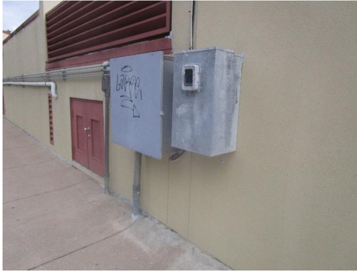
Figure 1 – Main Electrical Service and Meter.
