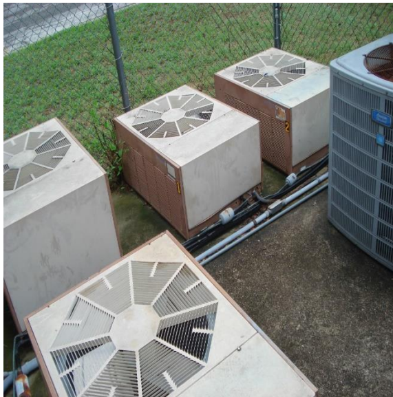
Figure 2 – Condensing Units
