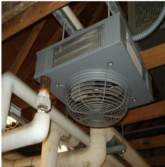
Figure 4 – Unit Heater with Corrosion at Pipe Connection
