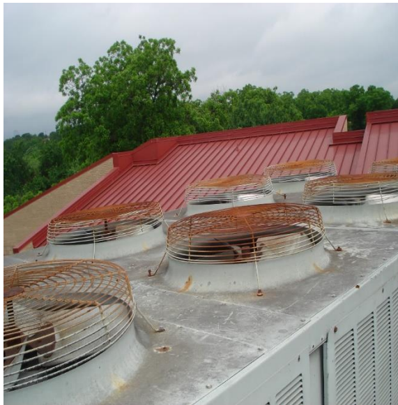
Figure 2 – Chiller Condensing Unit - Corrosion
