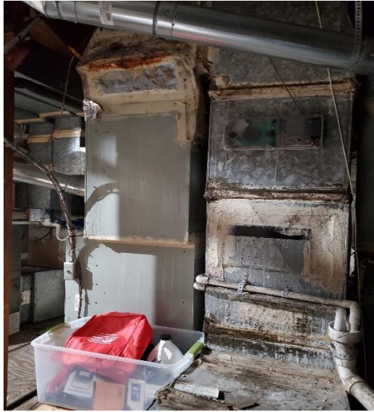
Figure 3 – Typical Ductwork with biological growth.
