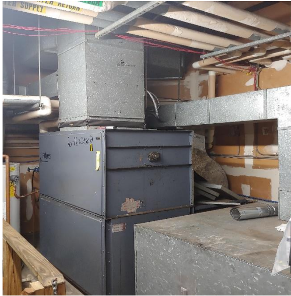
Figure 1- Typical AHU.
