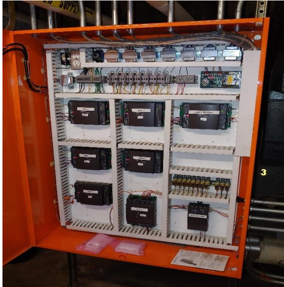
Figure 7 – Typical Controls Cabinet.
