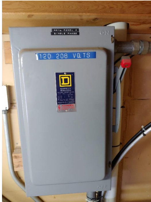
Figure 3 – Disconnect to Panelboard “A”.
