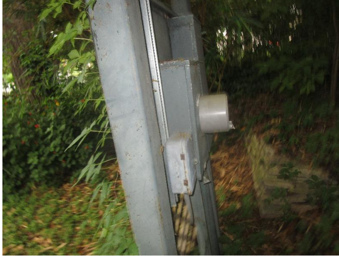
Figure 3 – Main Electrical Service in Courtyard.
