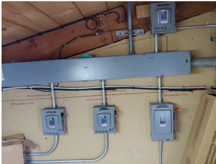
Figure 2 – Wireway in Mezzanine Mech/Elec Rm.
