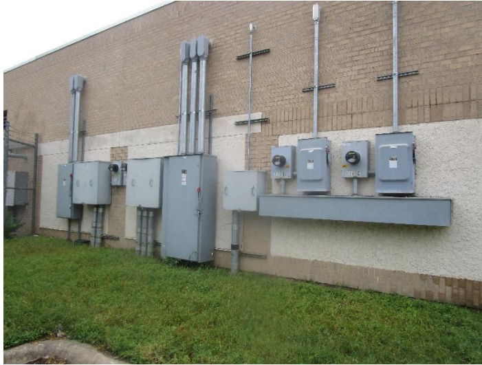
Figure 2 – Main Electrical Services.211A, 211B, 211C, & 211D
