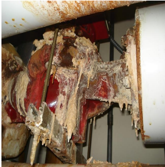
Figure 1 – Heating Water Pump Casing Corrosion
