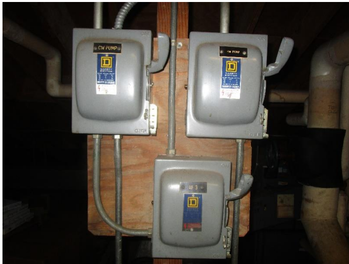
Figure 12 – Hot and Chilled Water Pumps disconnect switches
