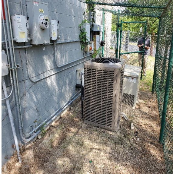
Figure 3 – Condensing Unit #1
