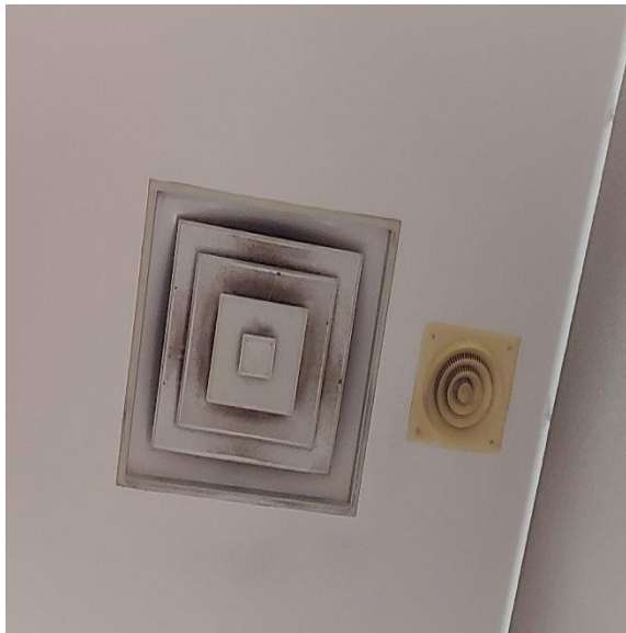
Figure 2 – Typical diffuser with rust, dirt and possible biological growth.
