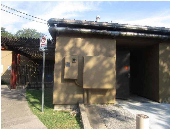
Figure 8 – Main Electrical Service CT enclosure and meter.
