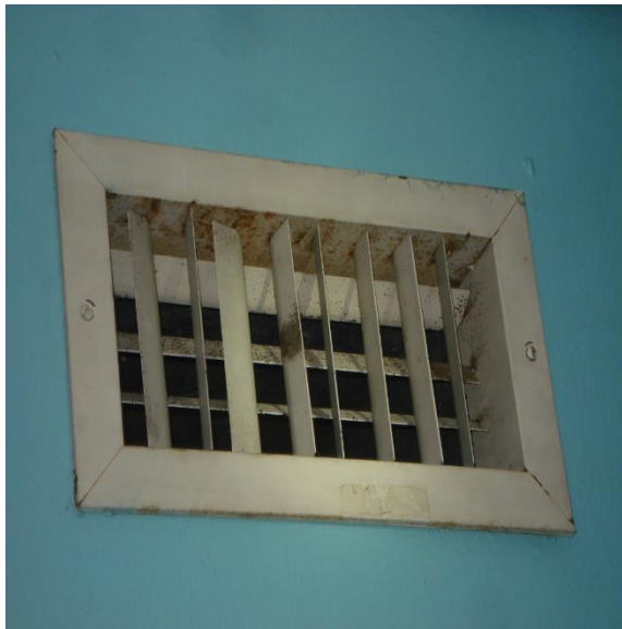
Figure 2 – Typical Air Device with Corrosion.
