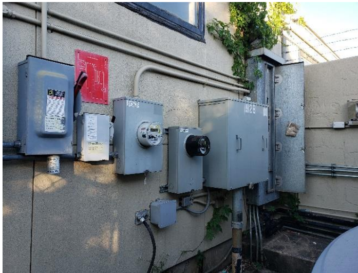
Figure 5 – Main Electrical Service in Mechanical yard.
