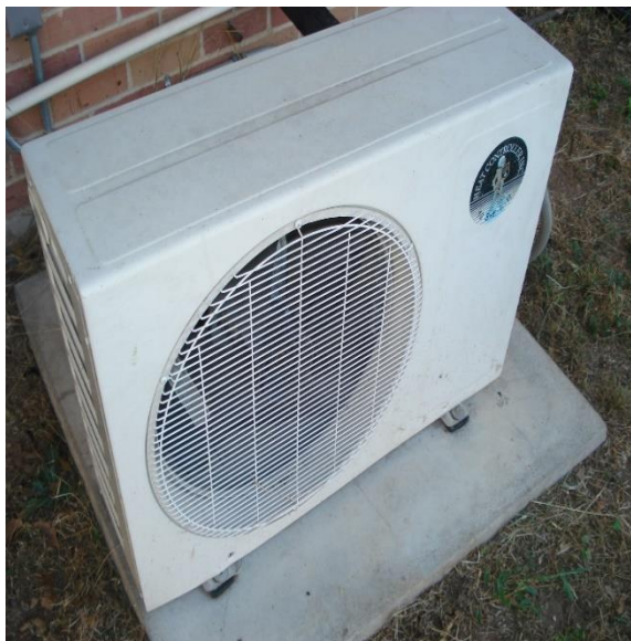
Figure 3 – Mini-Split condensing unit (typical of 3)
