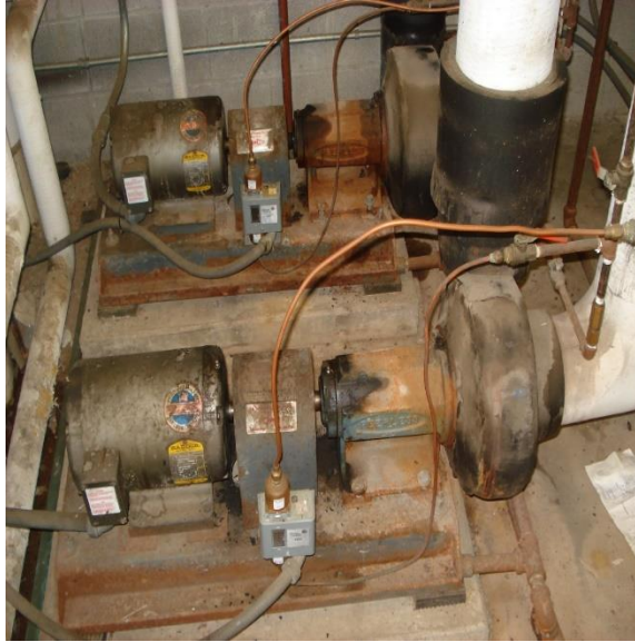
Figure 3 – Chilled water pumps
