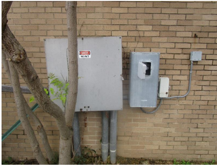
Figure 8 – Main Electrical Service and Meter
