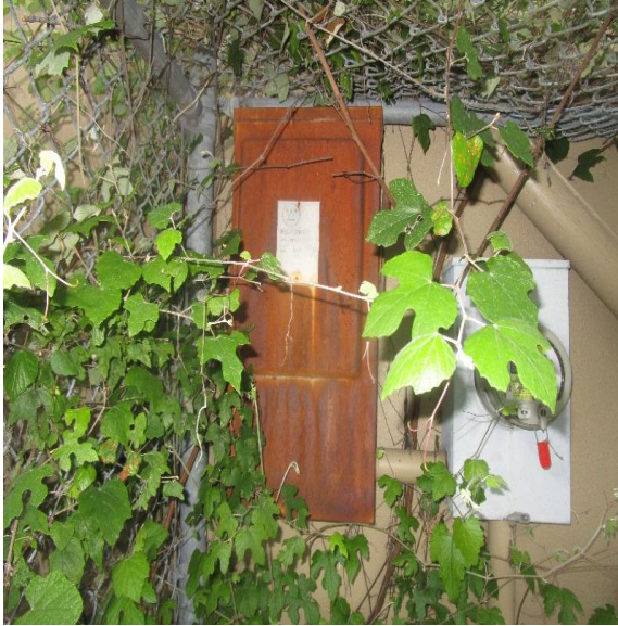
Figure 5 – Main Electrical Service Disconnect and Meter.
