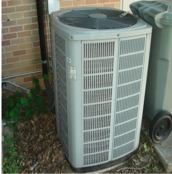
Figure 2 – AHU condensing unit (typical of 2)
