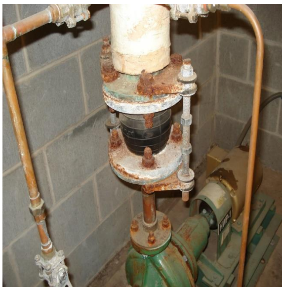
Figure 2 – Typical Pump with Corrosion
