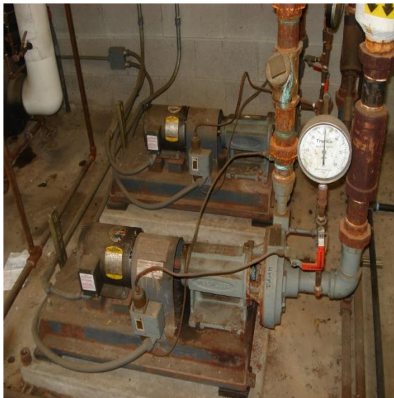
Figure 4 – Heating Water Pumps
