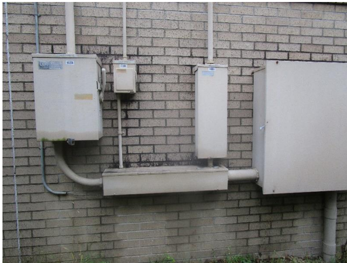
Figure 3 – Main Electrical Service in Electrical yard.
