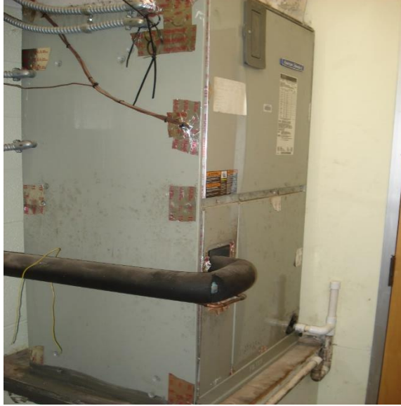
Figure 1 – ‘American Standard’ AHU
