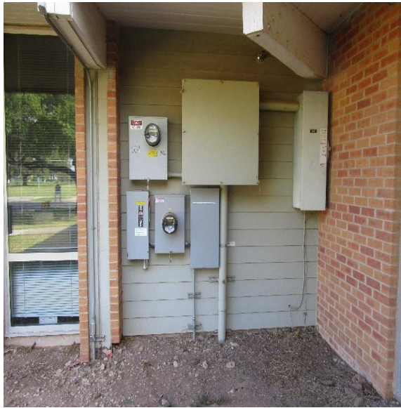
Figure 3 – Service Entrance and associated Metering
