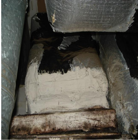
Figure 3 – AHU-1 Ductwork with biological growth.
