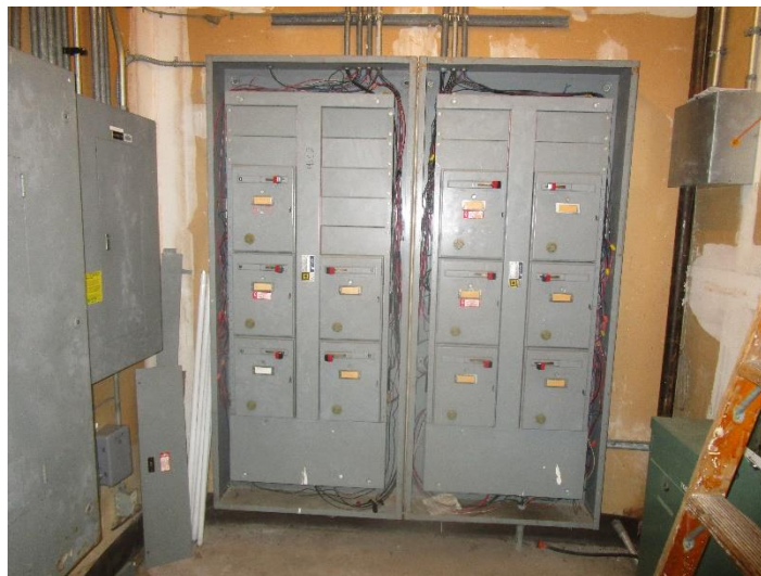
Figure 10 – Motor Control Center “MSC2”
