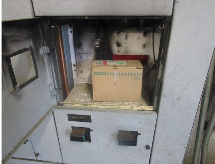
Figure 12 – MCC-1 Arc Flash Damage
