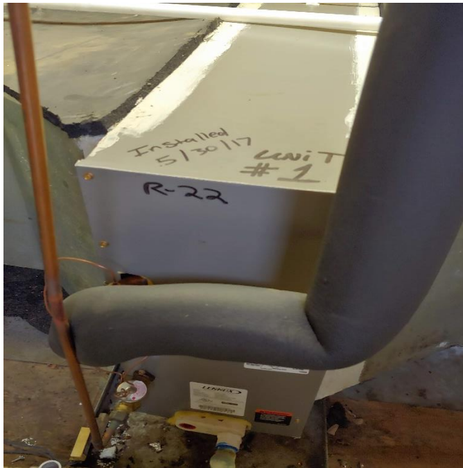
Figure 2 – AHU DX Cooling Coil (Typical 3 AHUs)
