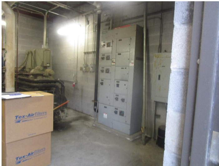
Figure 11 – Motor Control Center MCC-1
