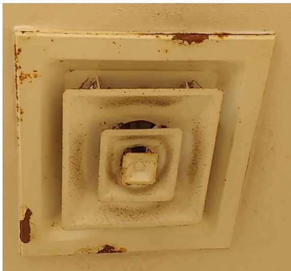
Figure 4: Typical Rusty Air Device with Suspected Microbial Growth
