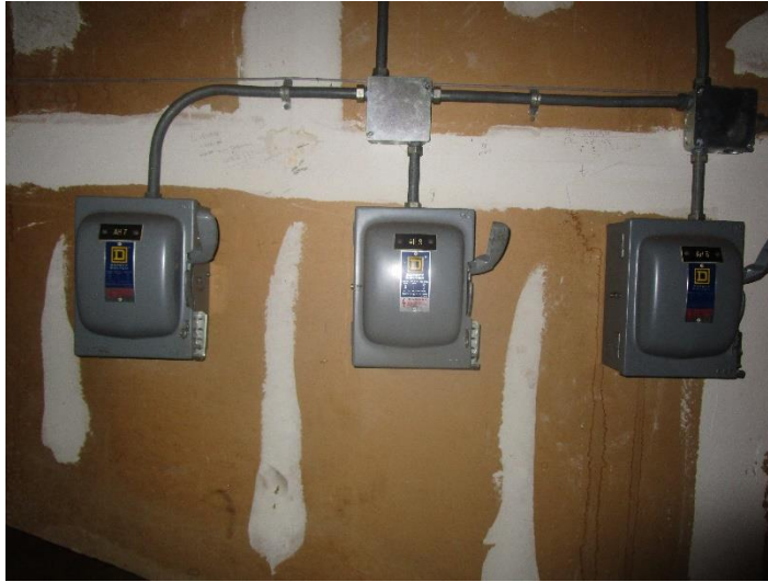
Figure 11 – Air Handling Unit disconnect switches
