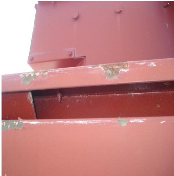
Figure 2 – ACCU-1 Corrosion on Condensing Unit Frame
