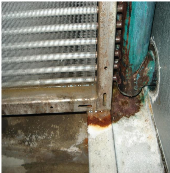
Figure 2 – Typical AHU Cooling Coil Corrosion
