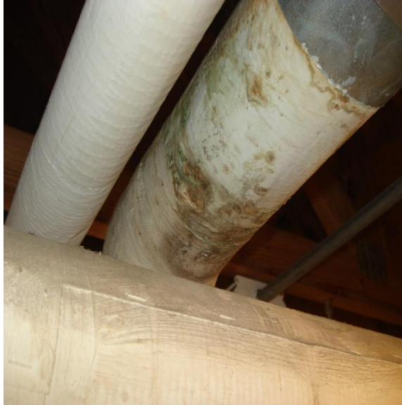
Figure 3 – Biological Growth and Water Damage on Pipe Insulation
