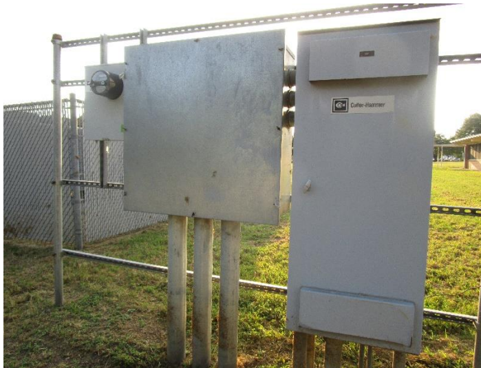
Figure 5 – Main Distribution Panel “MDP”
