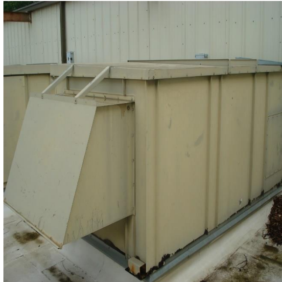
Figure 5 – Typical Roof Mounted AHU
