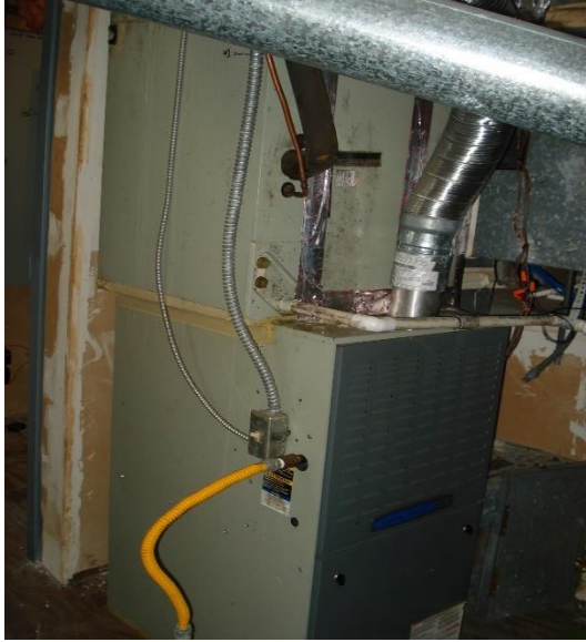
Figure 1 – AHU-1 (typical of all 3 AHUs)
