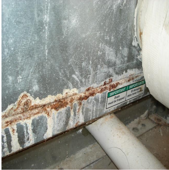
Figure 1 – Typical AHU Casing Corrosion
