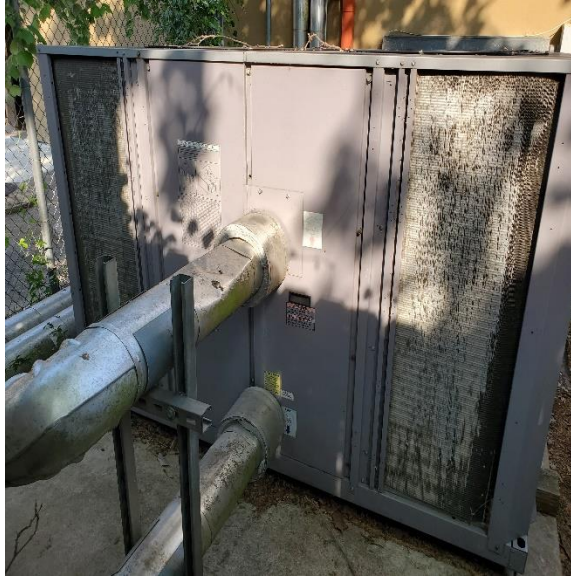
Figure 5 – Air-Cooled Chiller
