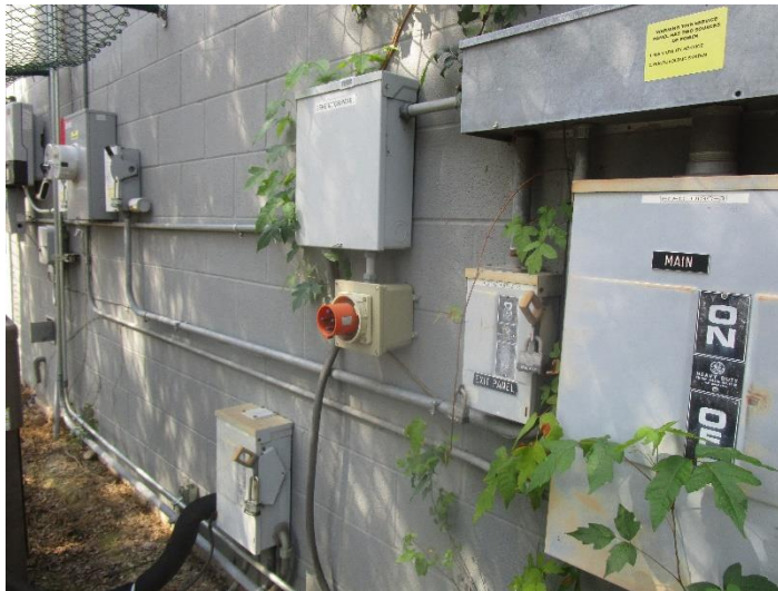
Figure 6 – Main Electrical Service and Disconnects.
