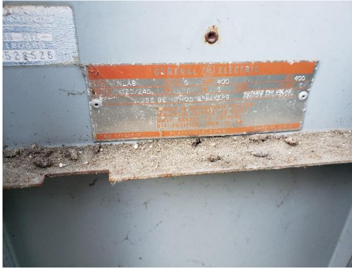
Figure 6 – Panelboard “MS-1” Nameplate & Debris
