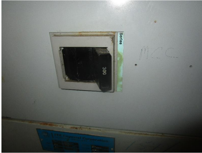
Figure 10 – Breaker to Motor Control Center “MCC-1”
