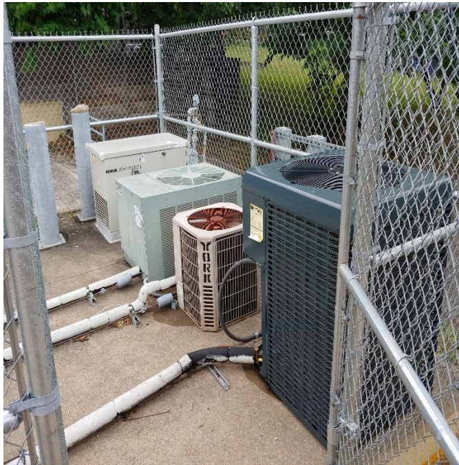
Figure 3 – DX Condensing Units and Generator
