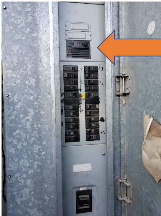
Figure 7 – Panelboard “MS-1” sub-feed breaker to Panelboard “A”.
