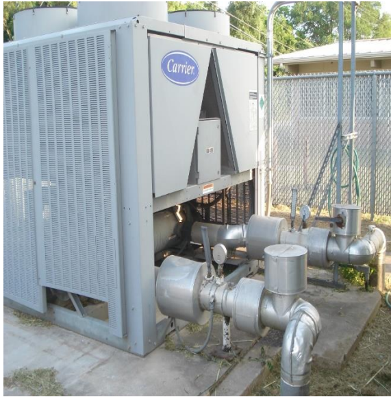
Figure 1 – Air Cooled Chiller and Exterior Piping
