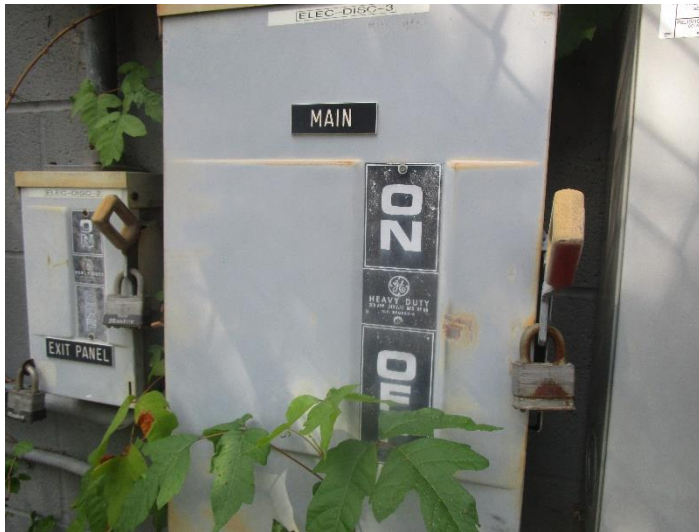
Figure 5 – Main Disconnect in Mechanical yard.
