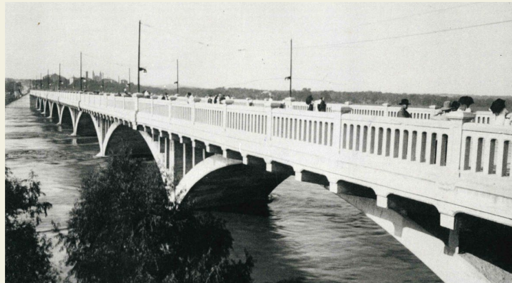
The 1910 original bridge was 50'-wide and carried a trolley line. In 1980 the bridge was substantially widened, and the above-deck features lighting and guardrails were changed to more highway-type elements.
