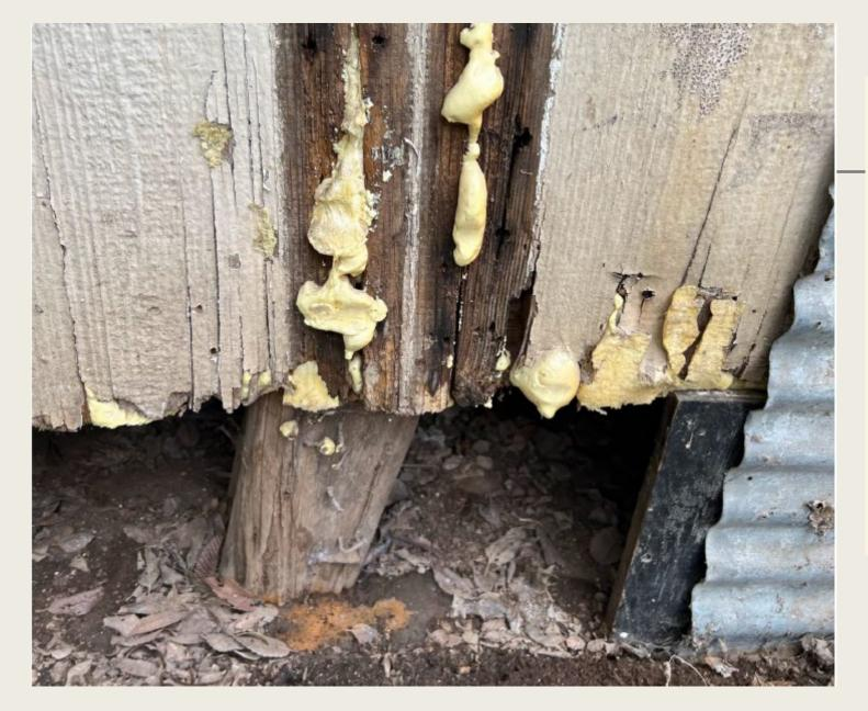
There are visible rotten and termite wood piers in multiple locations in the crawl space
