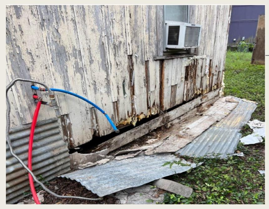
There is visible rotten wood on the framing members of the wall on the east and west side of the house.
