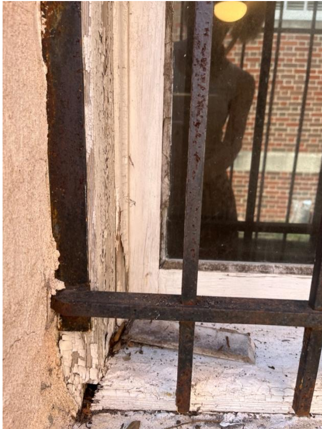
The first floor wood window has deteriorated over time and requires repair and repainting.
