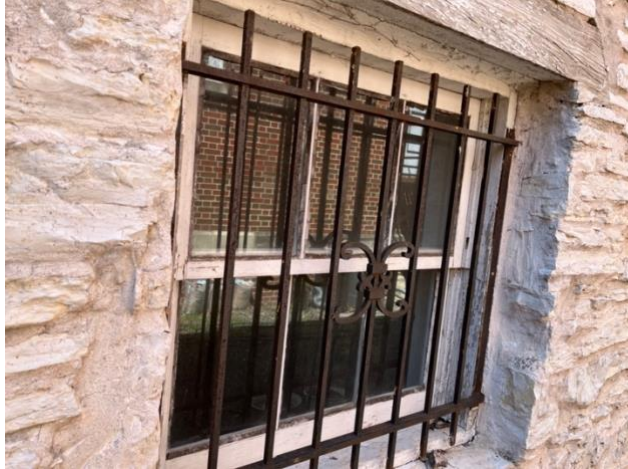
Detail of the first floor window, including wood rot at the bottom left corner.
