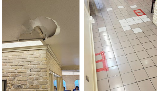
Damage to the center from AC Water Damage
