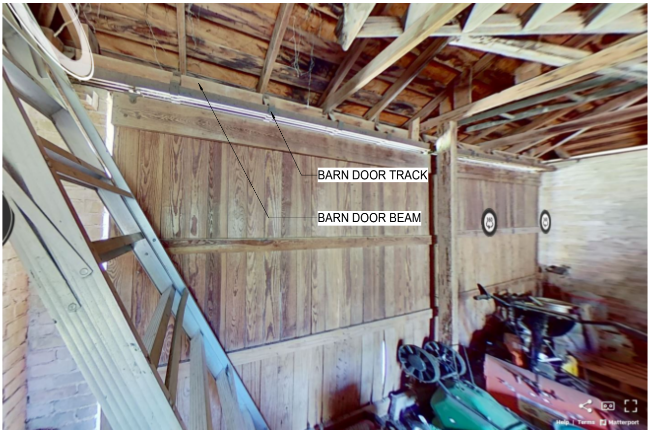
PHOTO 12: BARN DOOR, BEAM AND TRACK. DATE 2022-SEP-27.
