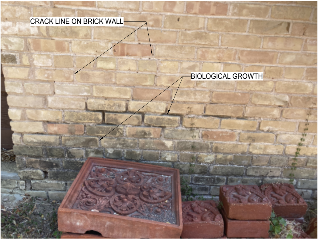
PHOTO 3: BRICK CRACKS AND BIOLOGICAL GROWTH ON SOUTH FACADE. DATE 2022-JUL-30.
