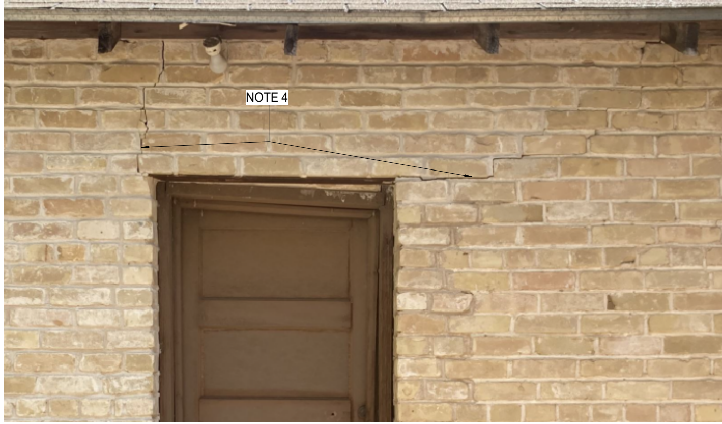
PHOTO 14: CRACKLINES ON SOUTH FACADE. DATE 2022-JUL-30.
