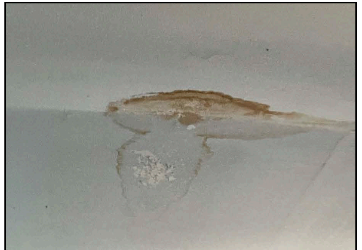
Ceiling leaks and mold
