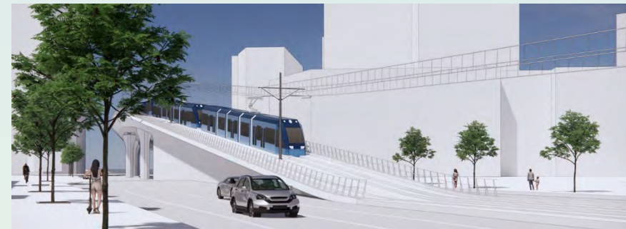
Retained Fill at West Riverside Drive
