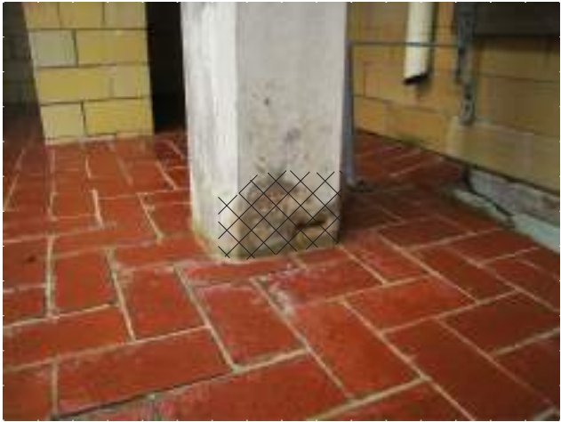
F COLUMN REPAIR x/x' = 1'-0"
