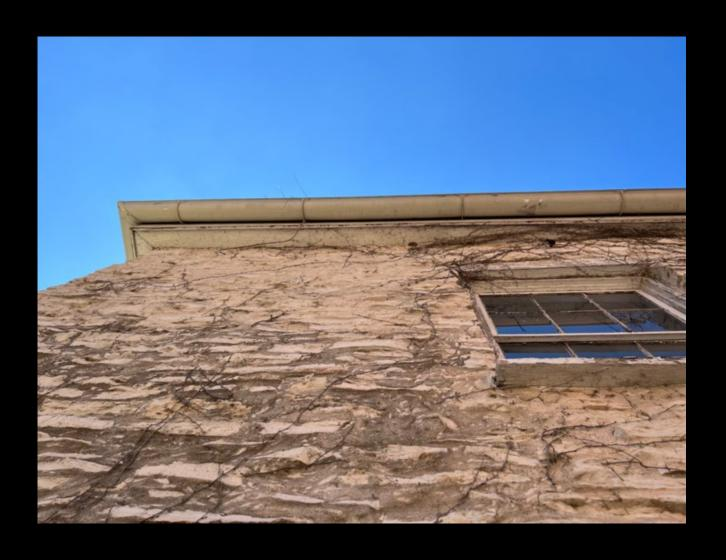
Wood fascia beneath the roof needs to be stripped and repainted to protect the original fabric.
