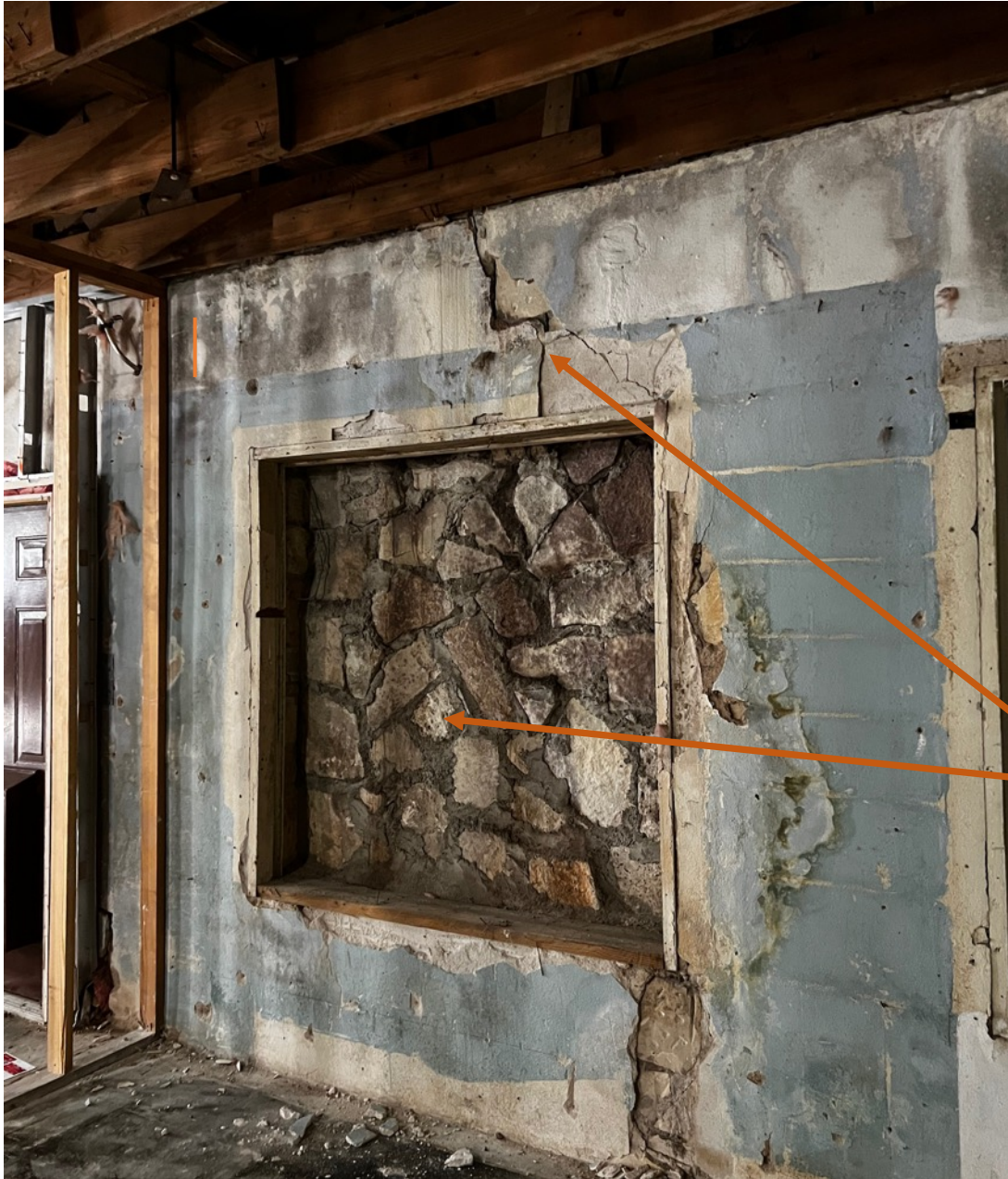
Interior view of window infill on south elevation
