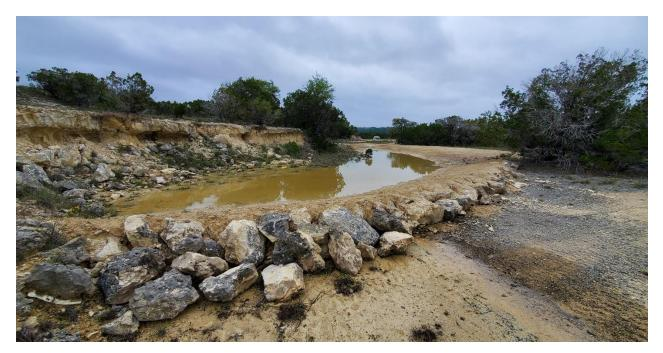
This newly installed conservation terrace on the Medway tract is part of an effort to restore a degraded area by reducing rainwater runoff and retaining water and soil on the landscape.
