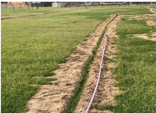
Current Construction of Irrigation Lines at Martin Multipurpose Fields
