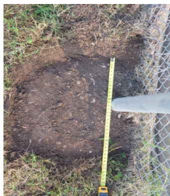
Photo of the Current 4' Deep Footing that is Supporting the Netting Poles The Footing will need to be Doubled to 8' to Accommodate the Increase in Height
