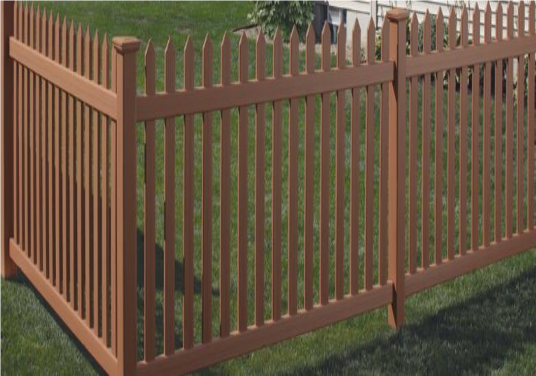
Gap between vertical members exceed 2" and potential for impalement
