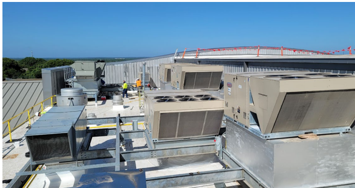
Cowan Elementary - High Efficiency HVAC Package Unit
