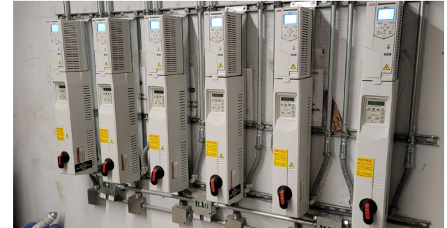
Rosedale School – New Classroom LEDs and Variable Frequency Drives on Hydronic Pumps
