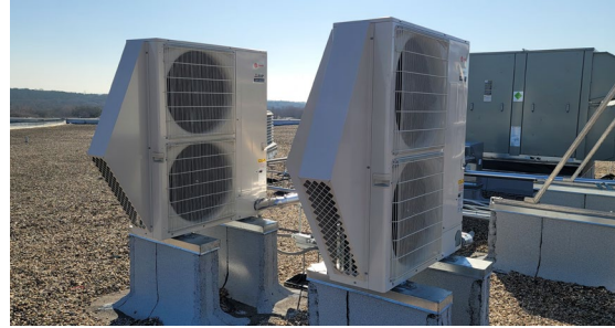
LBJ High School - Mini-split ACDX Heat pumps and HVAC package units
