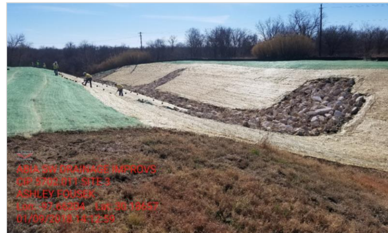
CIP Drainage Improvement Project (2018): Outfall 13 Erosion Repair and Stabilization Project (before and after photos)
