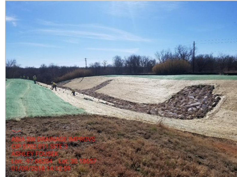
CIP Drainage Improvement Project (2018): Outfall 13 Erosion Repair and Stabilization Project (before and after photos)
