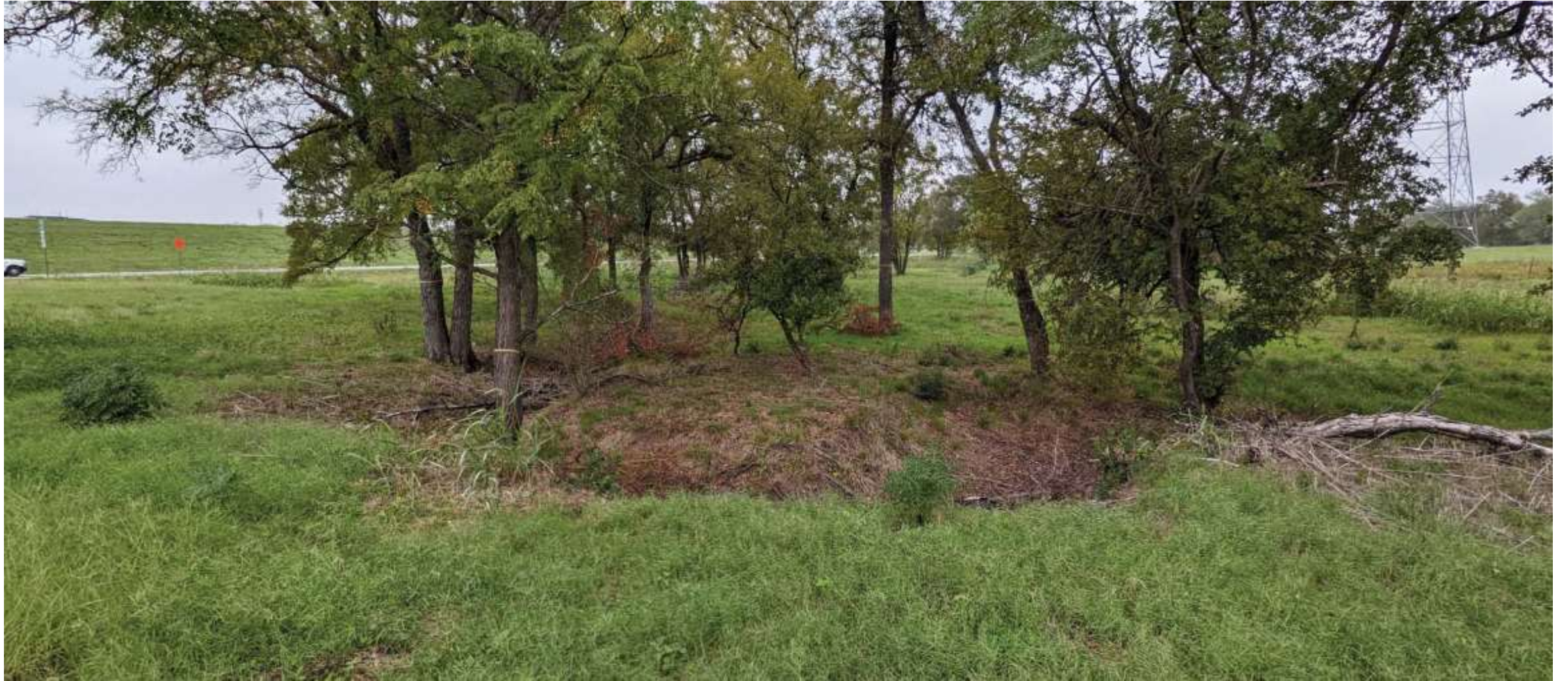
Highly eroded waterway.
