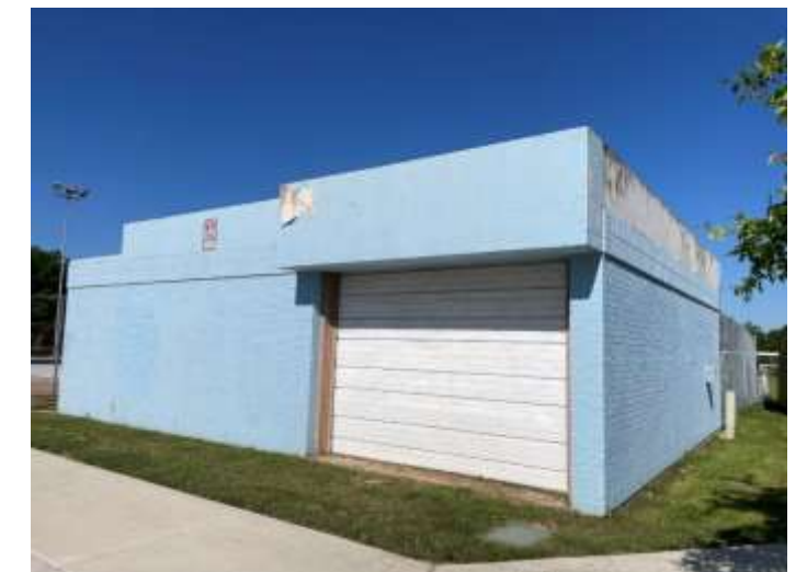
EXISTING RESTROOM – NORTHEAST
