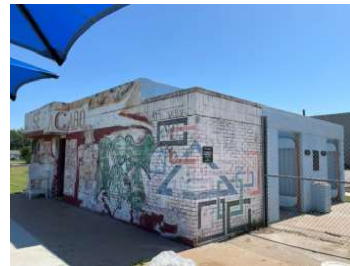
EXISTING RESTROOM – SOUTHWEST
