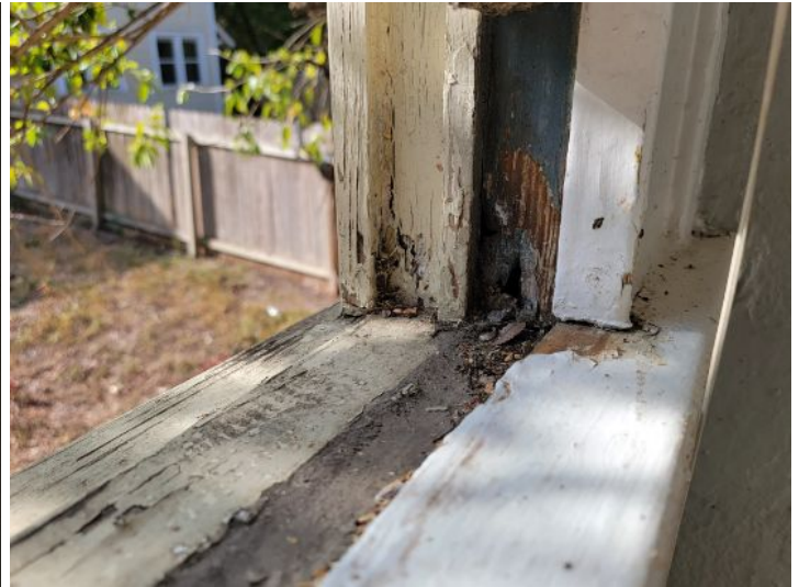
Deteriorated window frame
