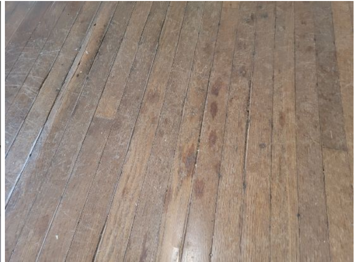
Deteriorated wood floors
