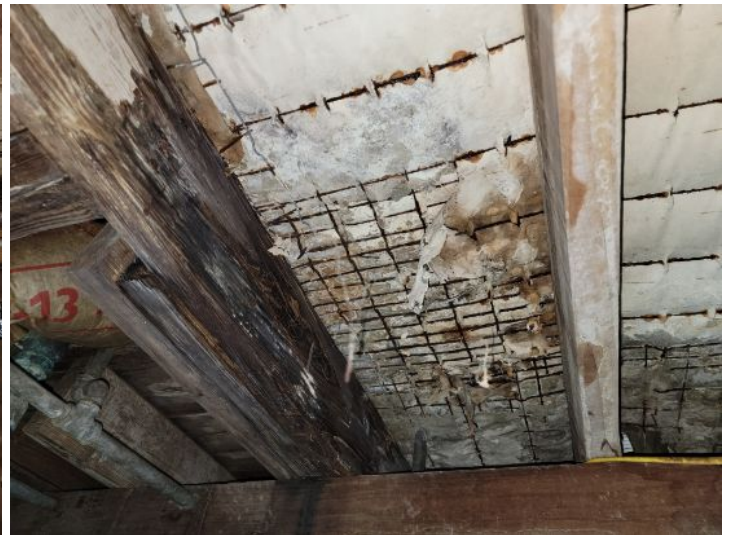
Moisture penetration in crawlspace
