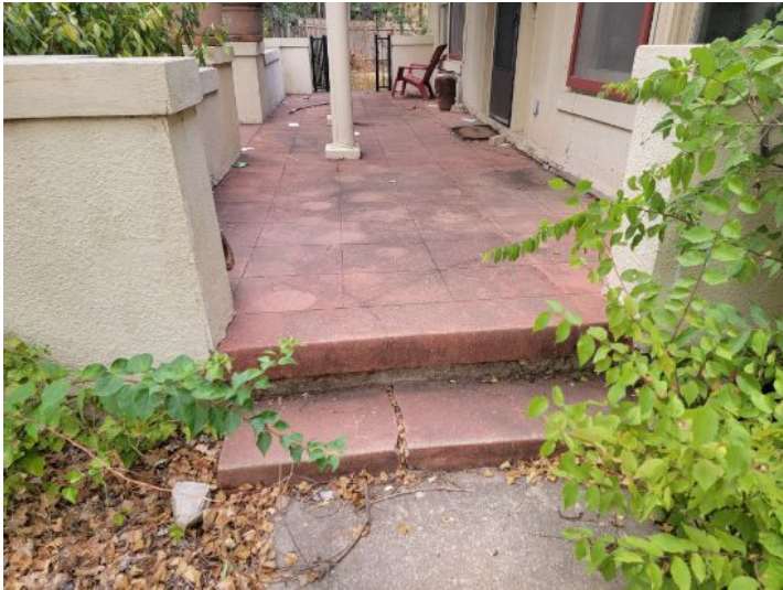
Cracking in front porch floor
