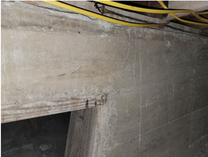
Cracking in foundation wall
