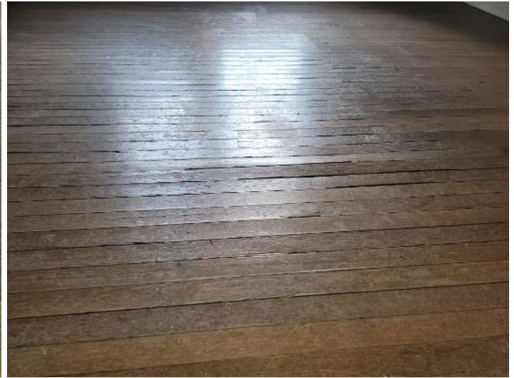
Loose and cupping wood floors
