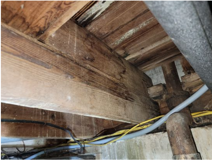
Basement: Evidence of moisture penetration and possible organic growth
