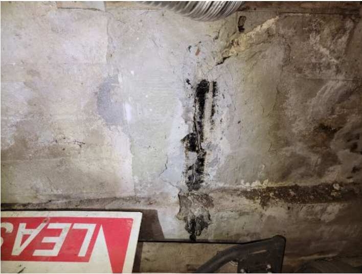
Cracking in basement foundation wall
