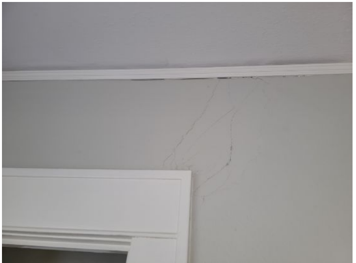
Cracking in wall
