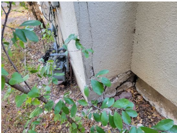
Cracking in stucco wall
