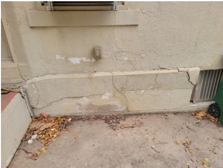
Cracking in foundation wall
