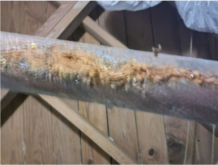
Corroded and rusted cast iron drain piping
