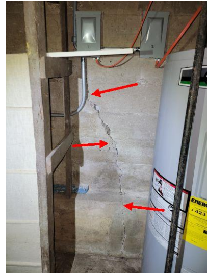
Severe cracking in basement foundation wall
