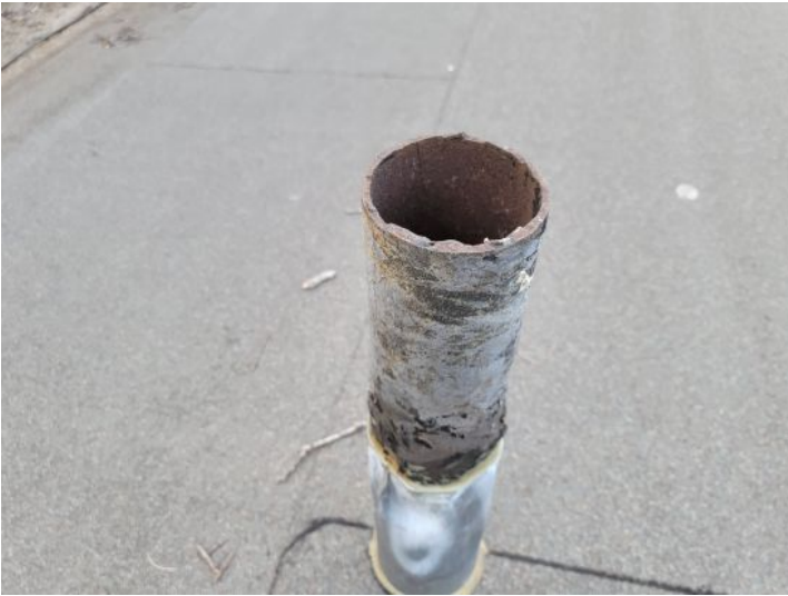
Improperly installed vent boot flashing
