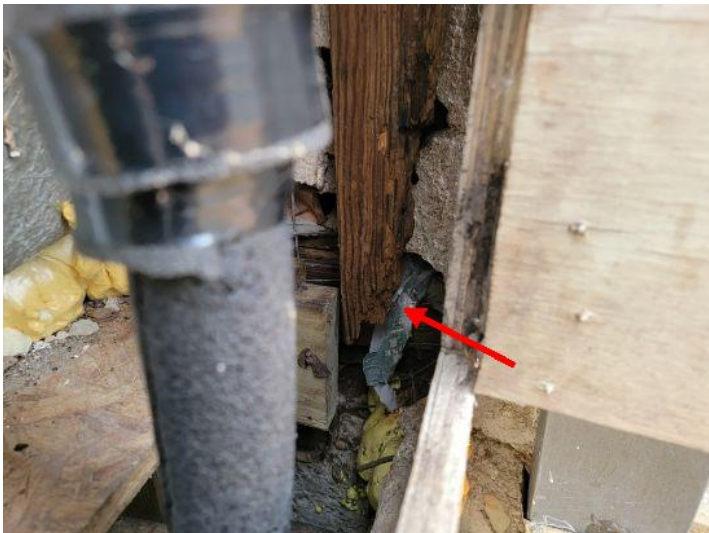
Deteriorated structural member
