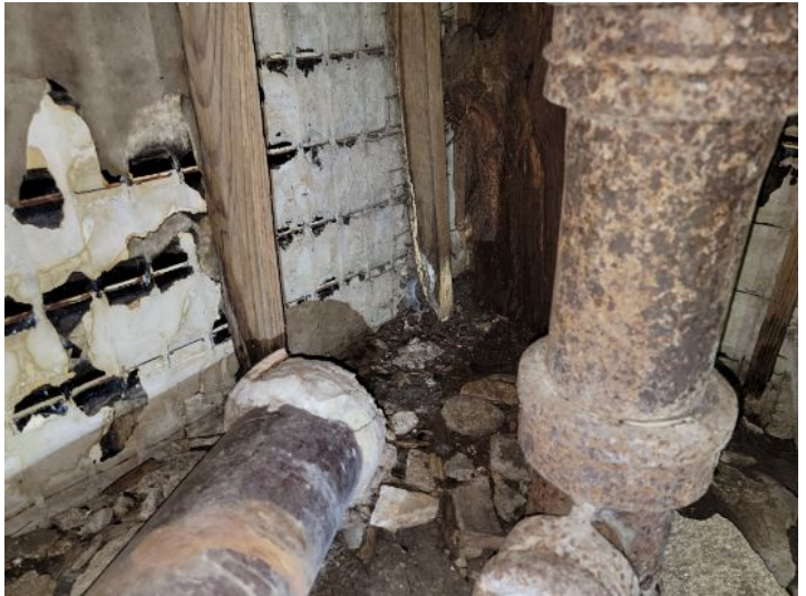
Crawlspace: Deteriorated structural support members
