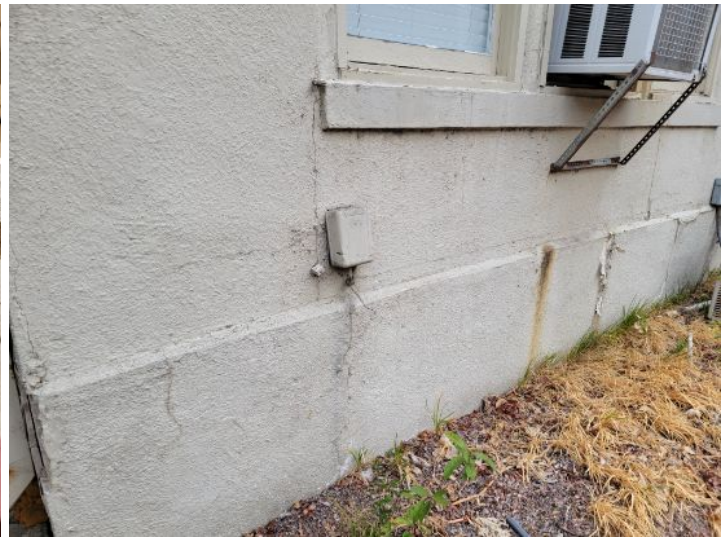
Cracking in stucco wall and foundation wall
