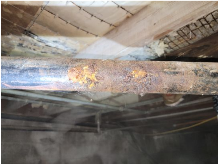
Rusted and corroded cast iron drain piping
