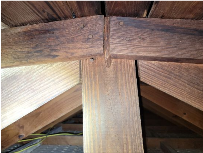
Gap in framing members. Water stains on decking and framing members.
