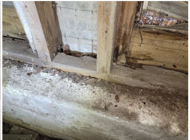
Crawlspace: Deteriorated structural support members
