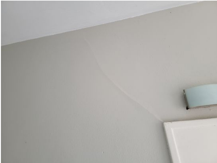
Repaired cracking in wall
