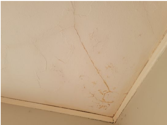
Cracking and water damaged ceiling
