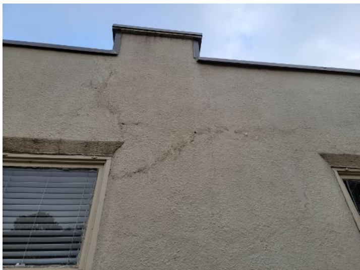
Cracking in stucco wall
