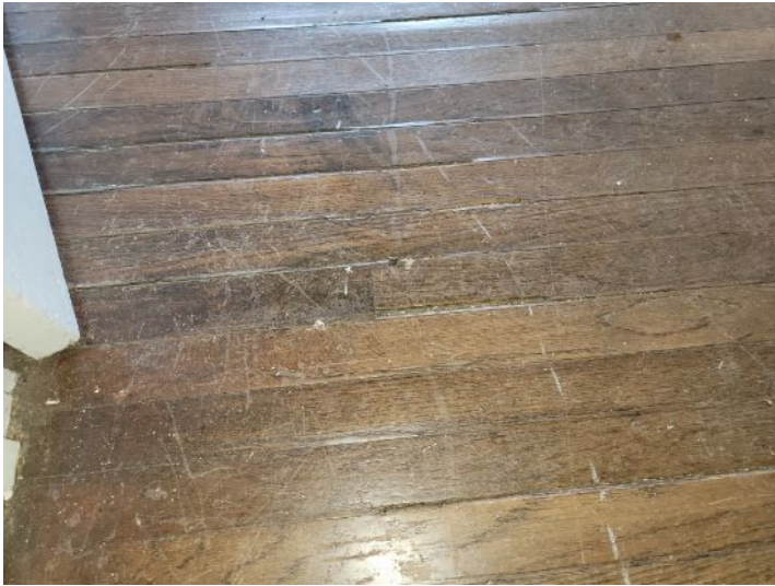
Deteriorated wood floors
