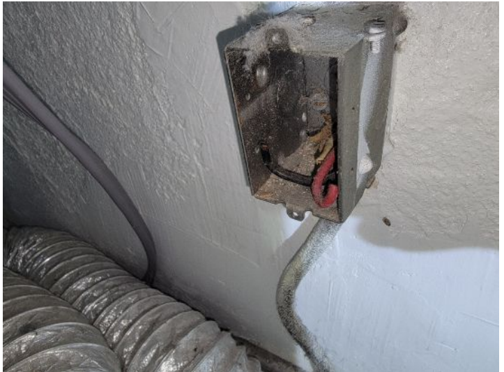
Missing conduit and cover
