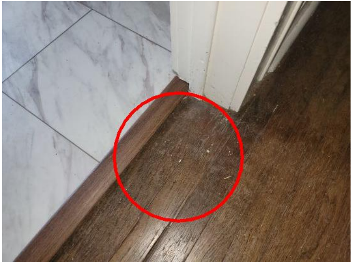
Evidence of wood destroying insect activity
