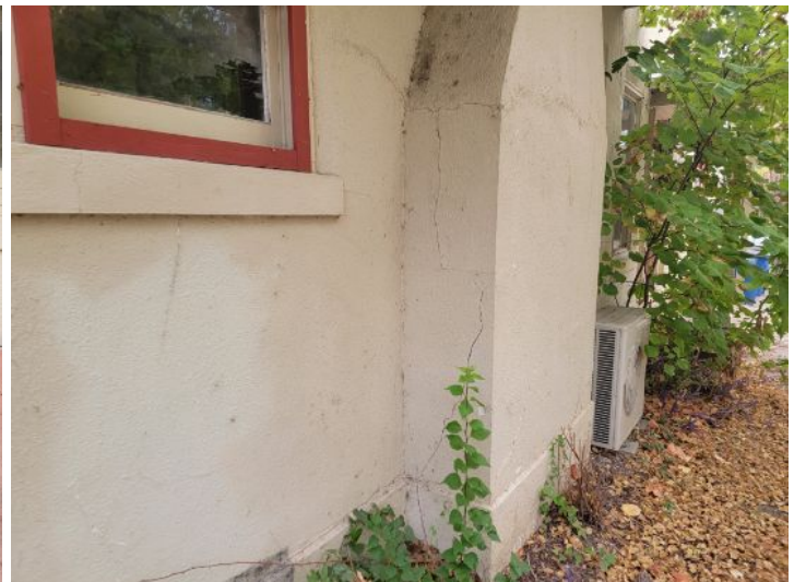
Cracking in stucco
