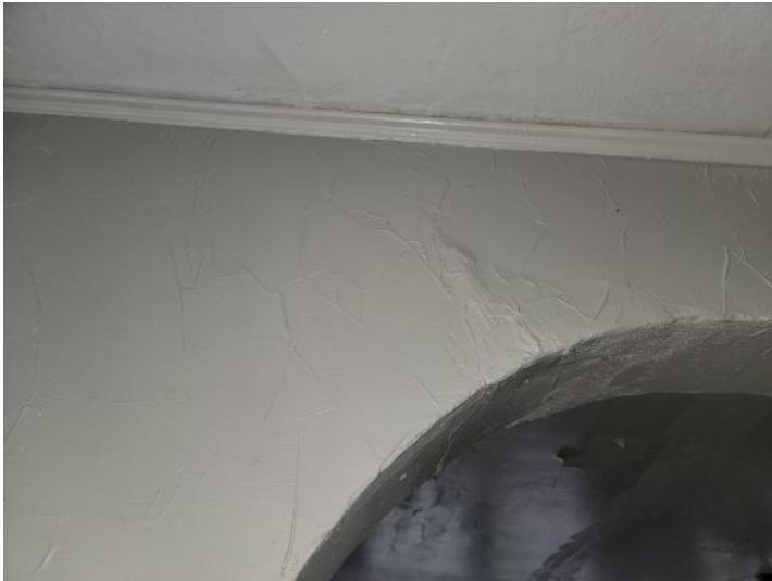
Repaired cracking
