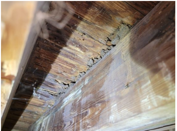
Evidence of wood destroying insect activity in basement
