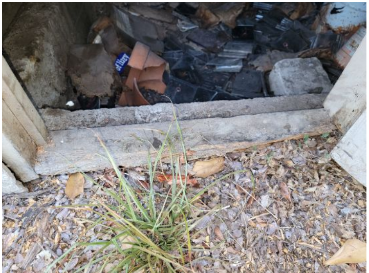
Wood to ground contact and deterioration.
