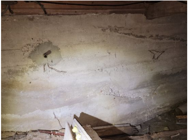
Cracking in foundation wall
