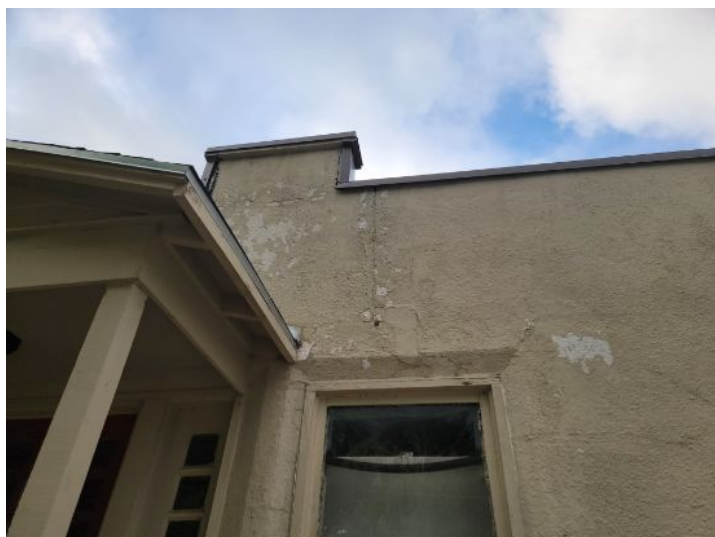
Cracking and flaking of stucco
