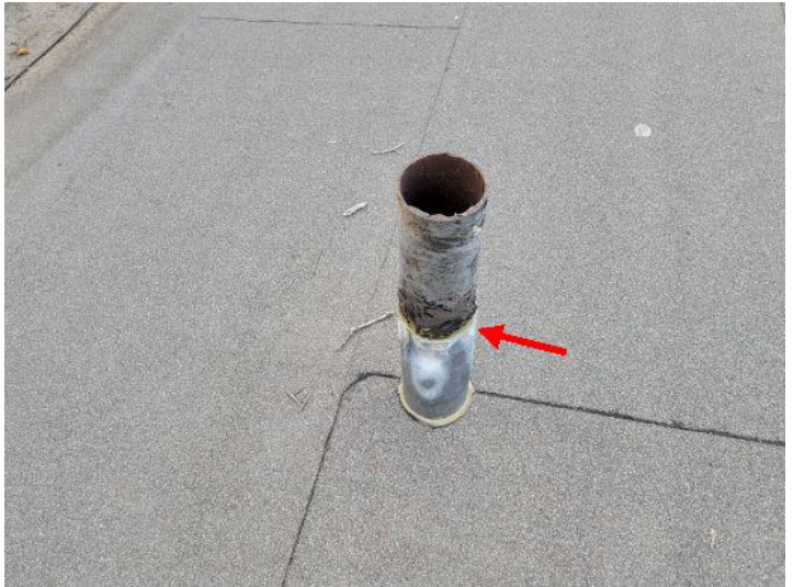
Improperly installed vent boot flashing
