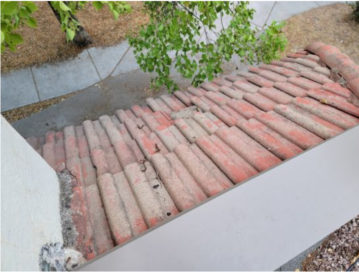
Cracked roof tiles
