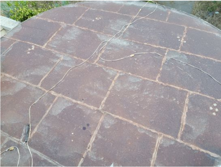
Rusted metal roof covering
