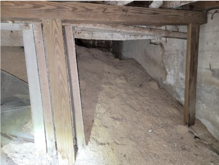
Crawlspace- wood to ground contact
