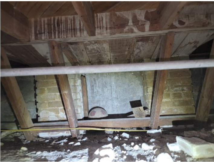
Wood to ground contact and possible organic growth
