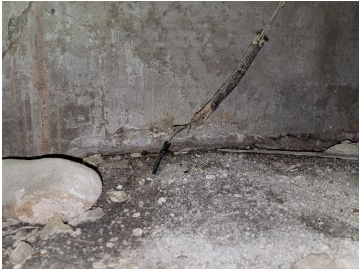
Damaged and exposed wiring
