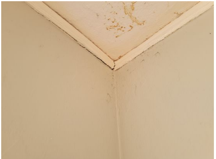
Water damaged ceiling and wall
