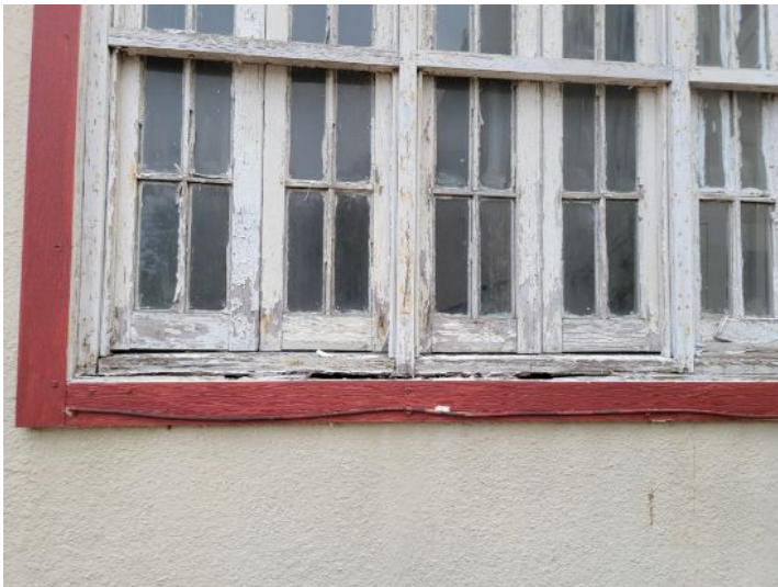
Deteriorated window frames
