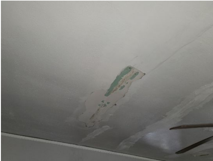
Evidence of moisture penetration
