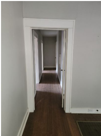
Door pass through out of square
