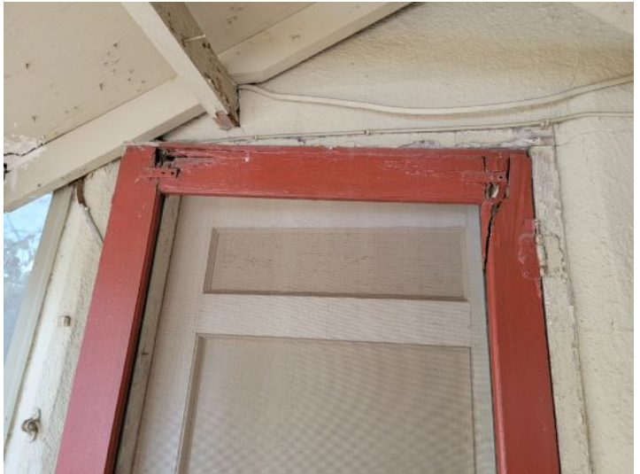
Deteriorated door
