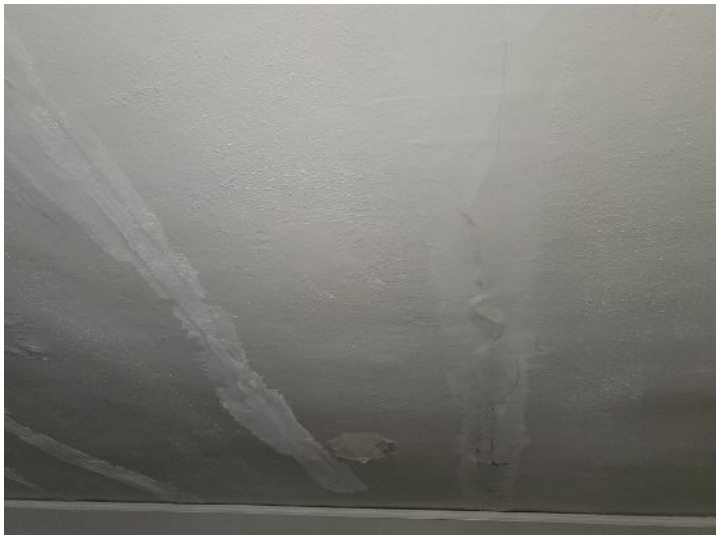
Evidence of moisture penetration
