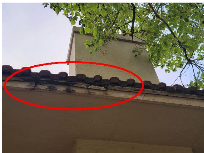
Deteriorated fascia
