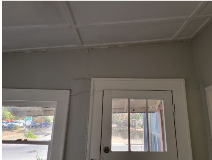
Cracking in wall
