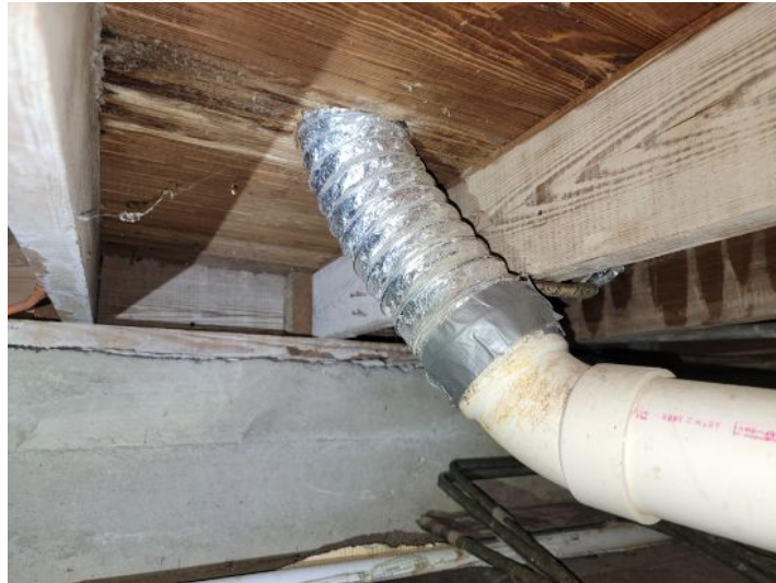
Improper dryer exhaust duct
