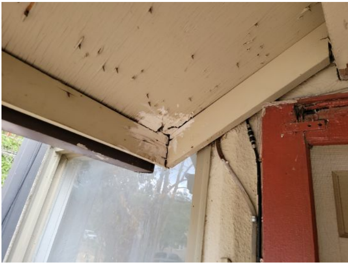
Deteriorated roof decking
