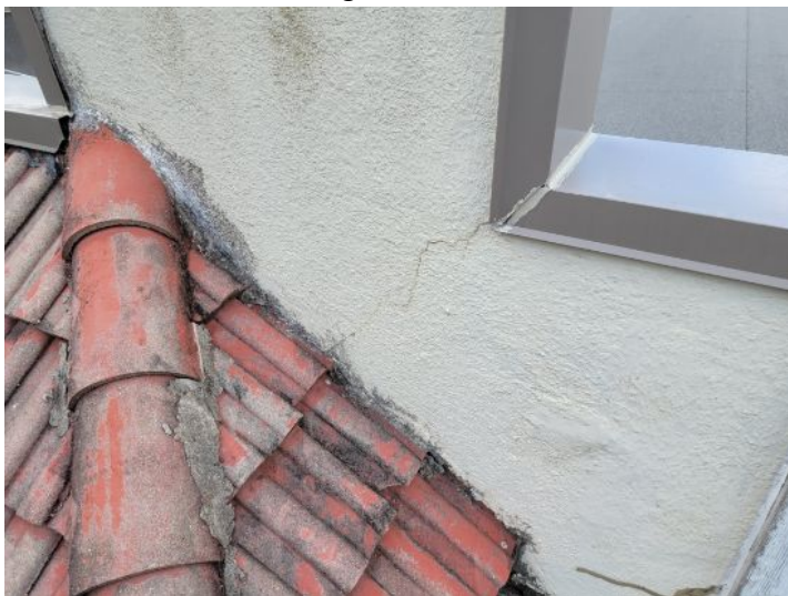
Cracking in stucco wall
