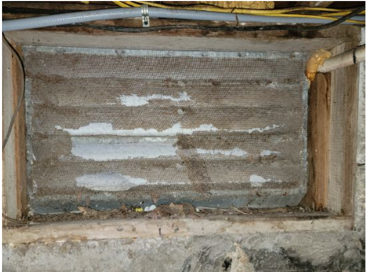
Damaged basement vent screen and evidence of moisture intrusion into basement
