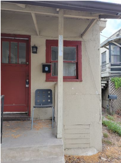
Bowed and warped support post
