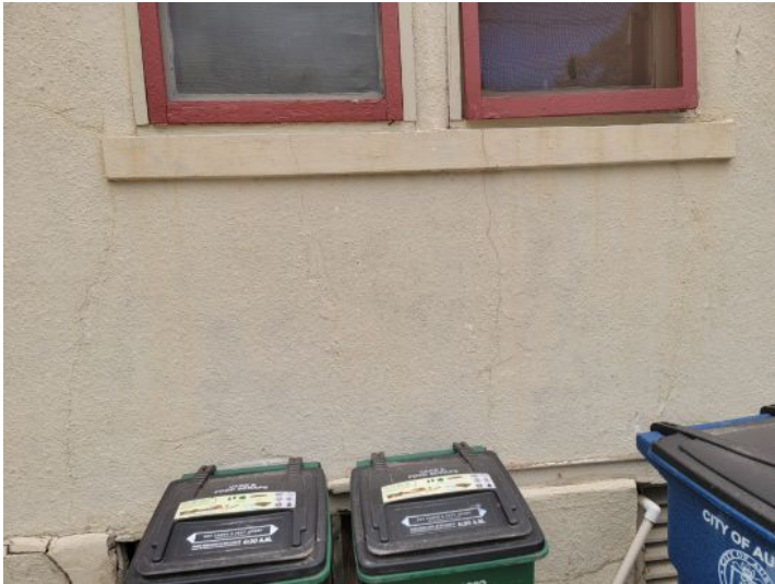
Cracking in stucco
