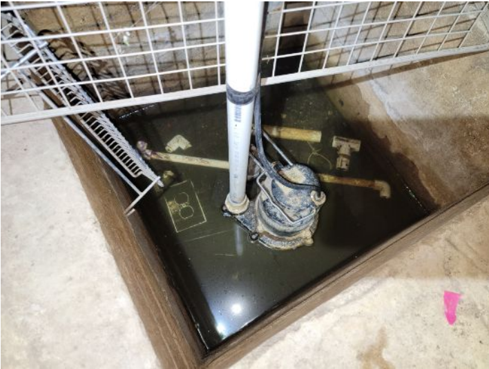
Sump pump well full of water and debris
