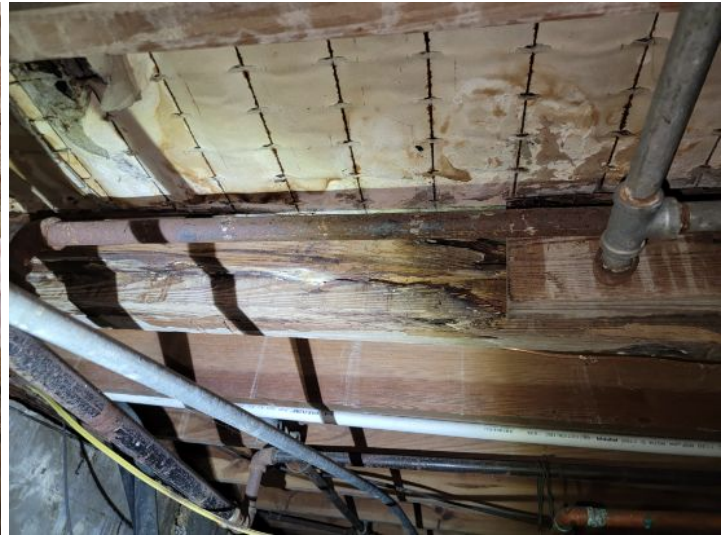
Deteriorated floor joists and sub-floor
