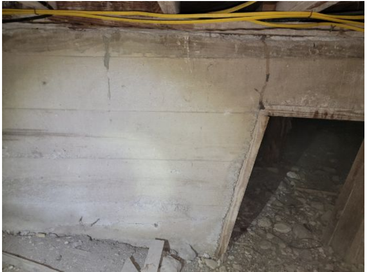
Cracking in foundation wall
