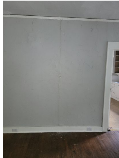
Cracking in wall
