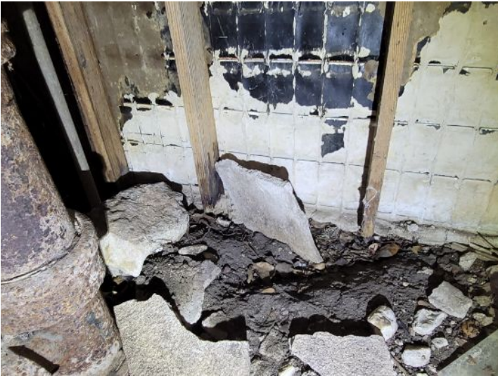
Crawlspace: Deteriorated structural support members
