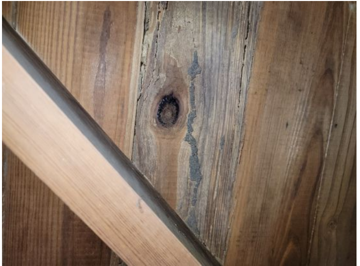
Evidence of wood destroying insect activity in crawlspace
