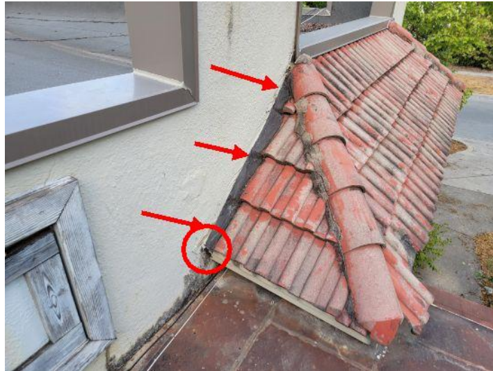
Improperly flashed sidewall and missing kickout flashing
