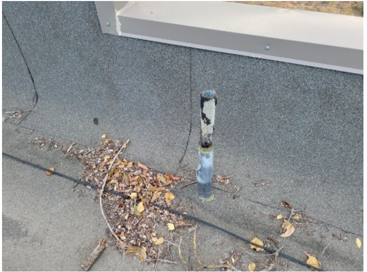
Improperly installed vent boot flashing
