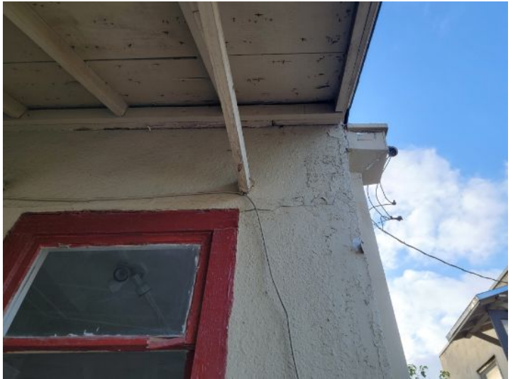
Cracking in stucco wall
