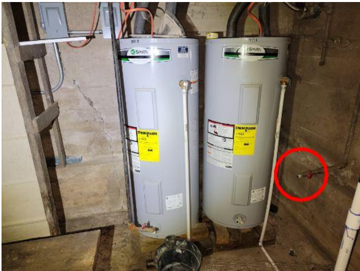
Water heaters and uncapped gas line
