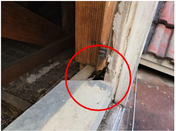
Deteriorated framing members
