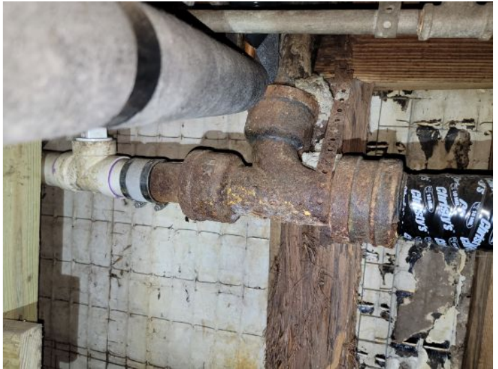
Corroded and rusted cast iron drain piping
