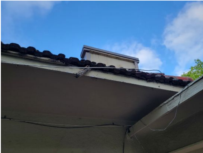
Deteriorated fascia
