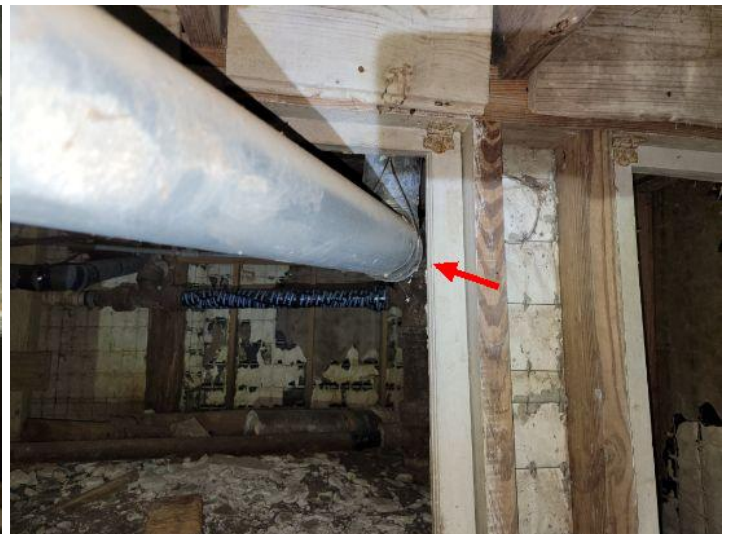
Inadequate clearance
