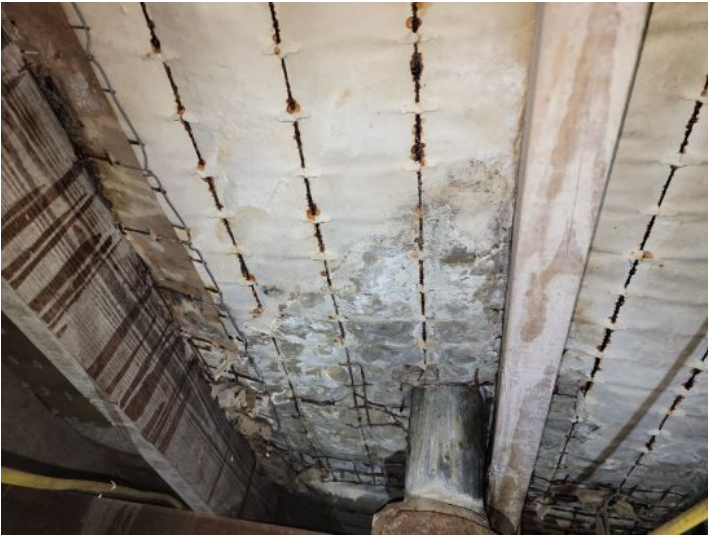
Evidence of moisture penetration and possible organic growth in crawlspace
