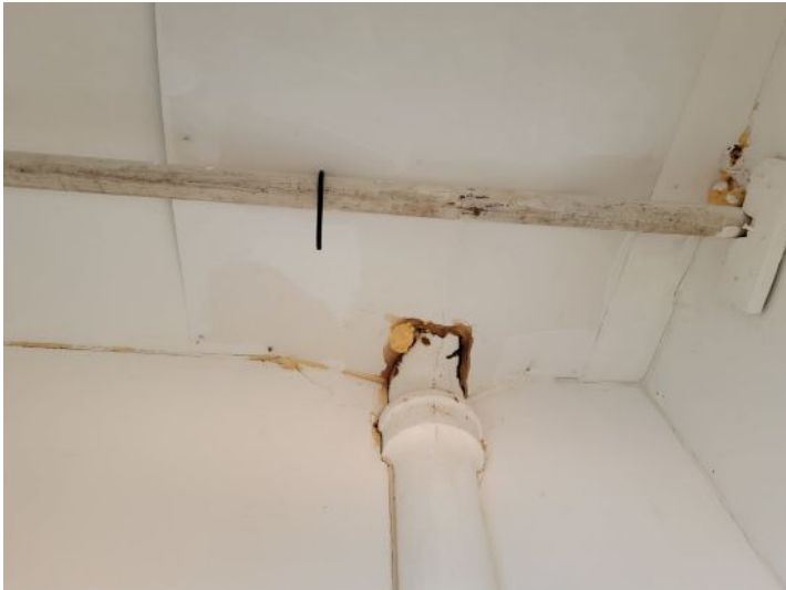
Water damaged ceiling and wall
