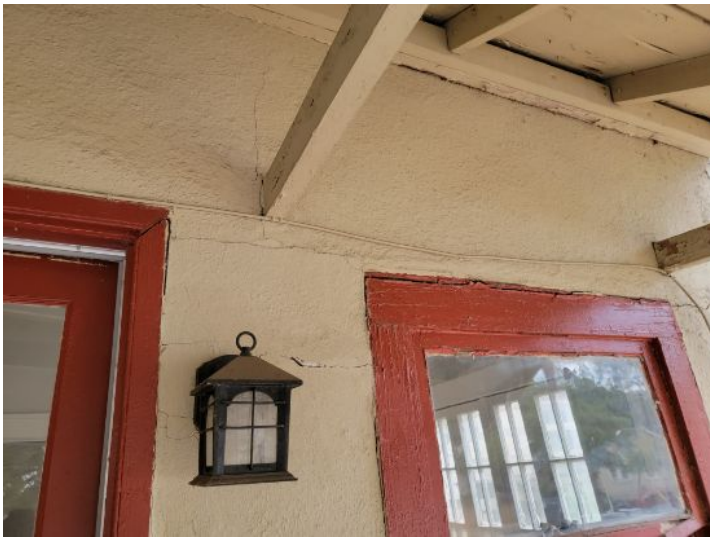
Cracking in stucco wall
