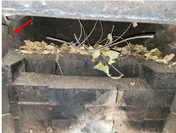
Cracking and debris in firebox/flue
