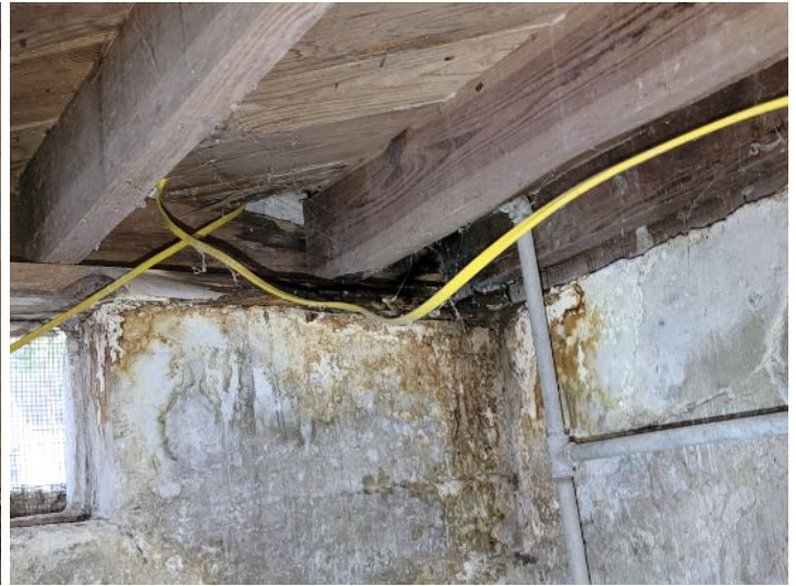
Deteriorated sub-floor members in crawlspace
