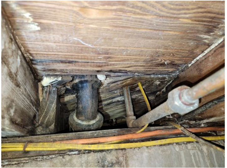
Basement: Sub floor deterioration and moisture penetration
