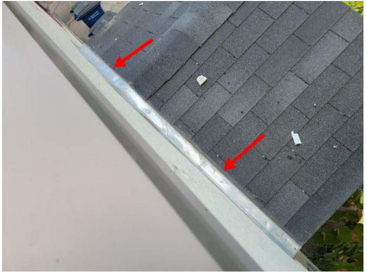
Improperly flashed headwall
