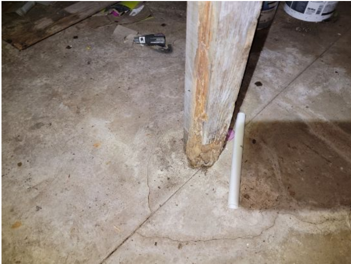
Rodent damaged basement support post
