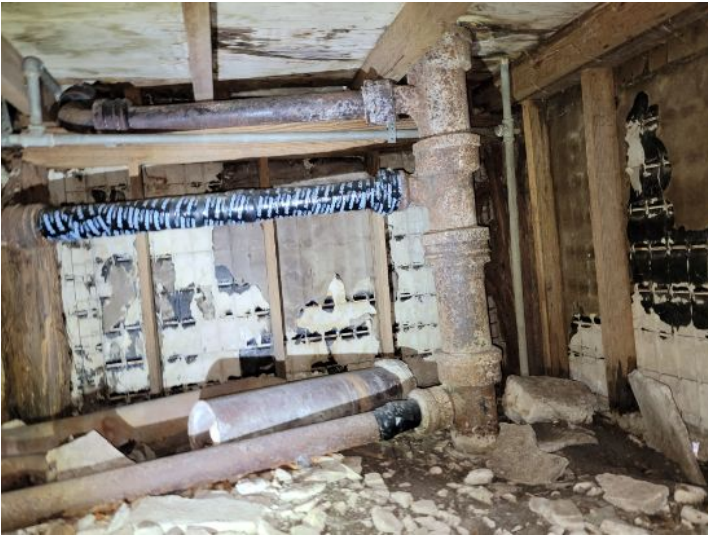
Corroded and rusted cast iron drain piping
