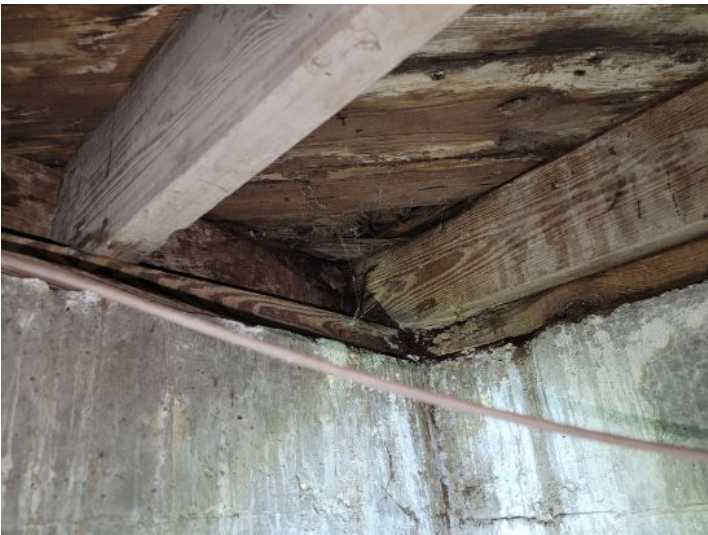
Deteriorated sub-floor members
