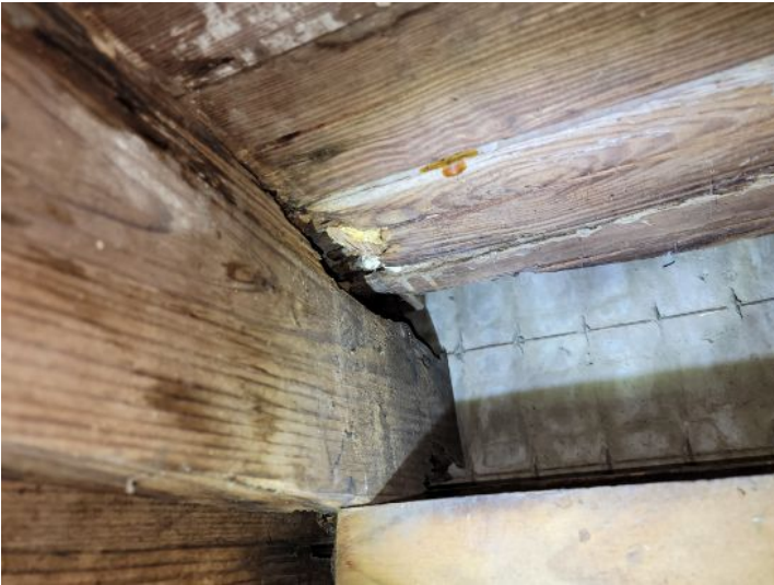
Deteriorated sub-floor and joist in crawlspace
