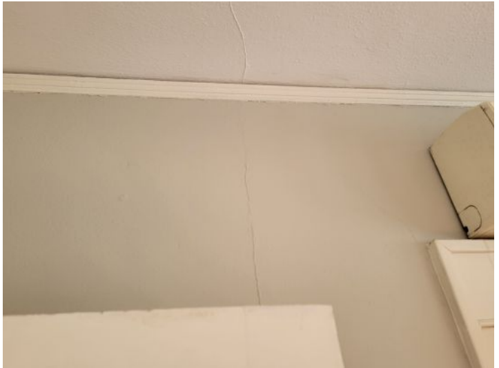
Cracking in ceiling and wall
