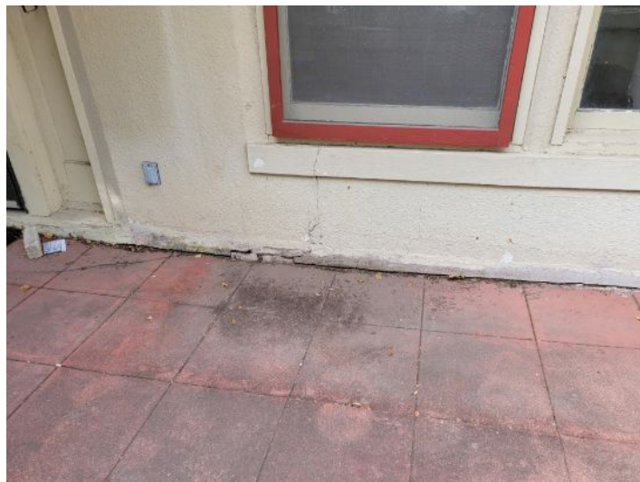
Front porch sloped towards the structure
