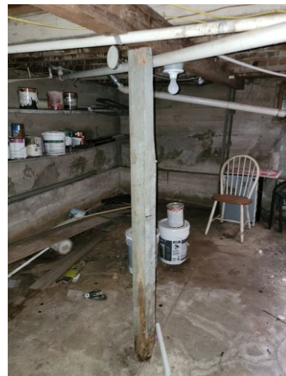
Rodent damaged basement support post
