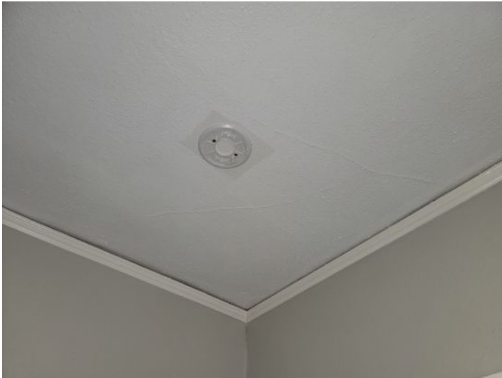
Cracking in ceiling
