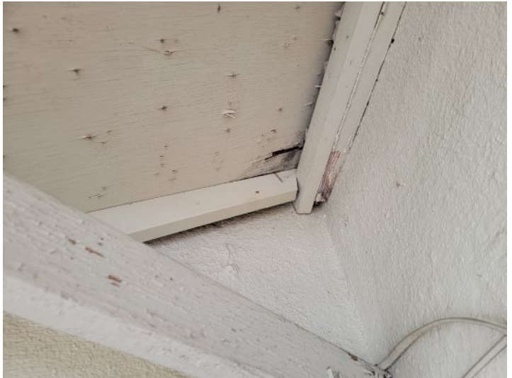
Deteriorated roof decking
