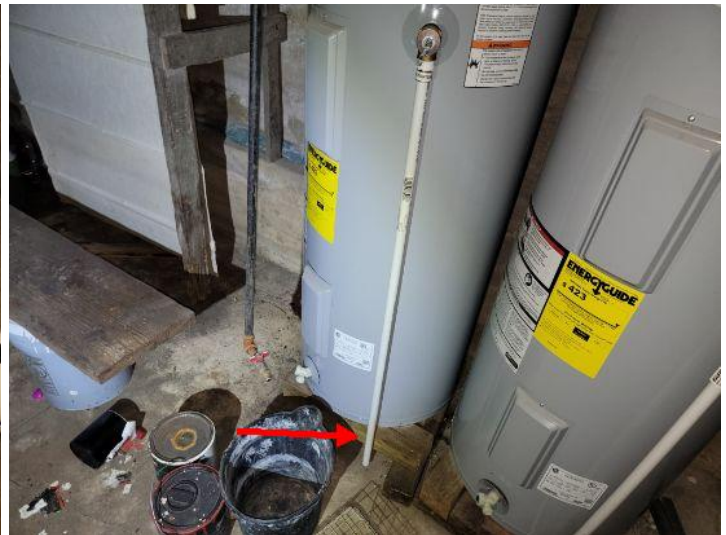
Improperly terminated TPR valve
