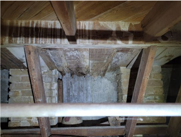
Deteriorated and fallen sub-floor
