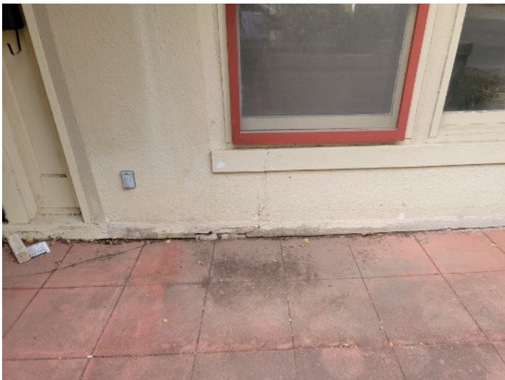
Cracking in stucco
