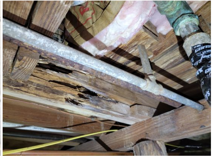
Deteriorated floor joists
