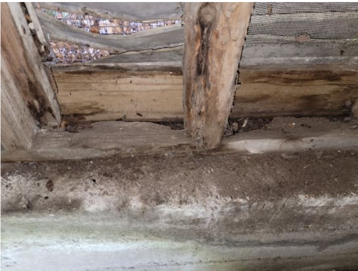
Crawlspace: Deteriorated structural support members
