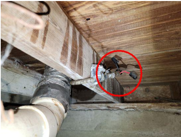
Improperly terminated wiring
