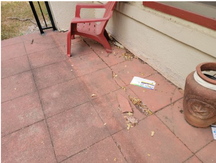
Cracking in front porch floor
