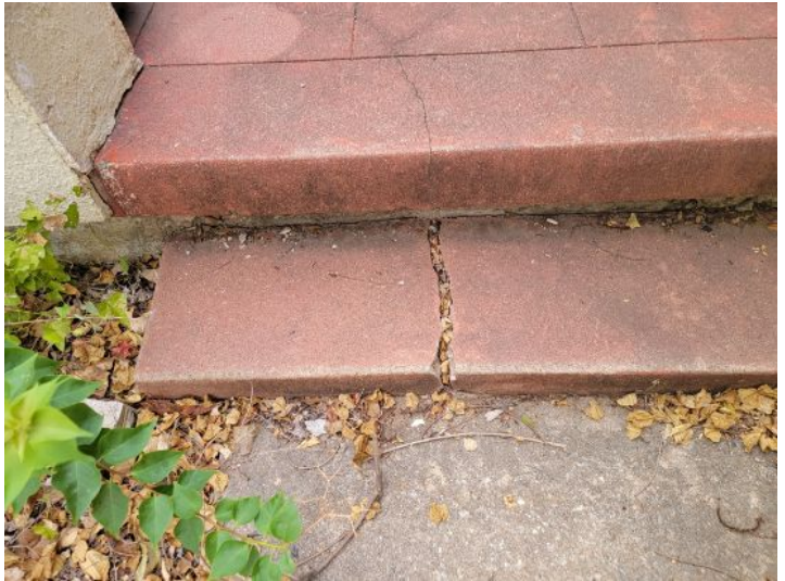
Cracking in front porch floor
