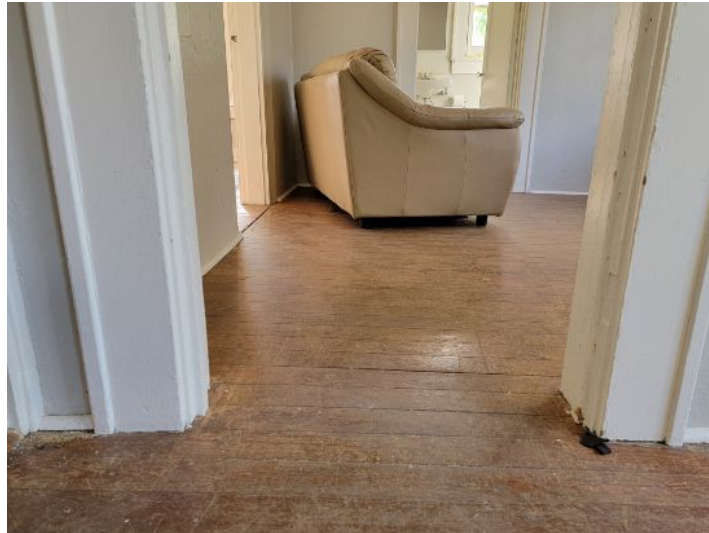
Severely unlevel floor
