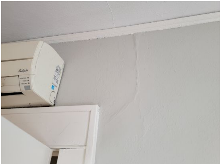
Repaired cracking in wall
