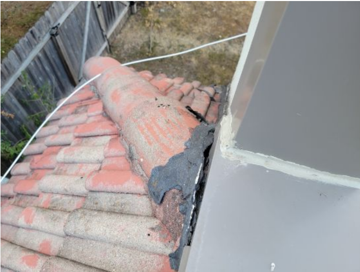
Damaged roof tiles
