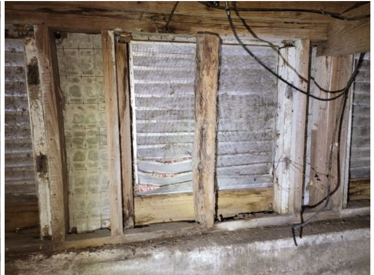
Crawlspace: Deteriorated structural support members
