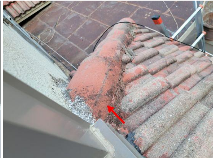
Cracked roofing tile
