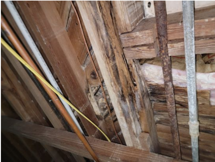
Deteriorated floor joists and sub-floor
