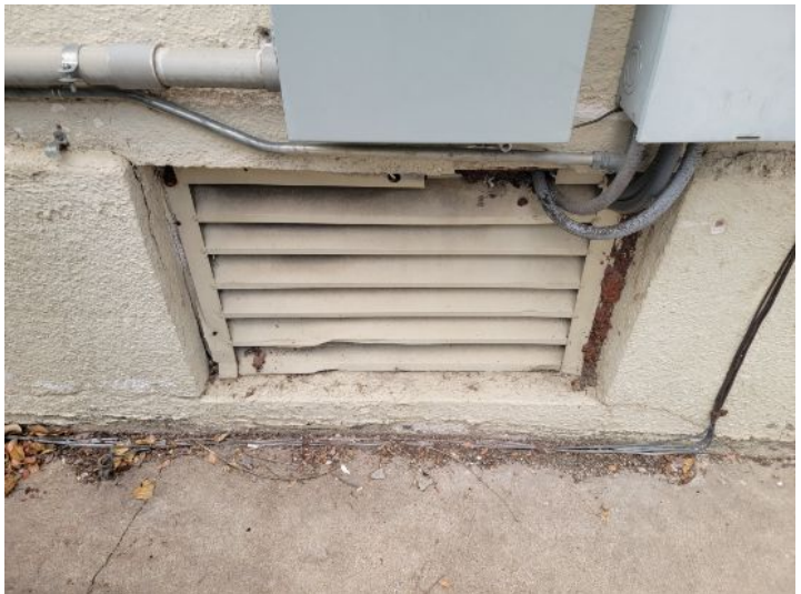
Damaged vent louver
