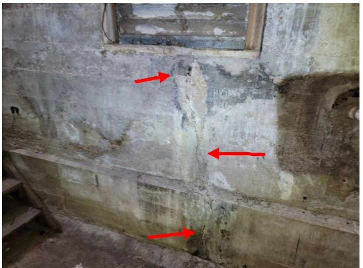
Severe cracking basement foundation wall
