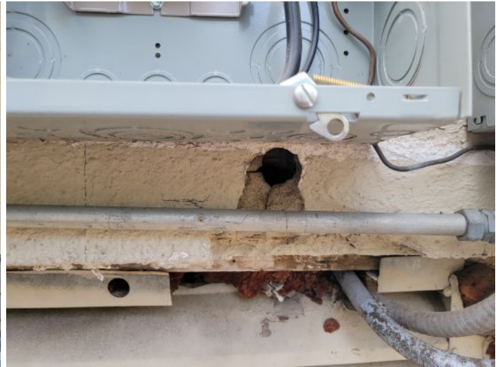
Hole in exterior wall
