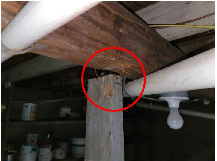
Disconnected basement support post
