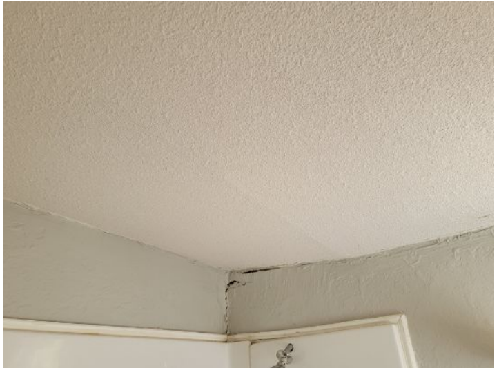
Sagging, damaged, and out of plumb and unlevel ceiling in 3013 Unit
