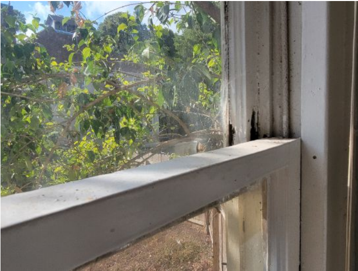
Deteriorated window frame
