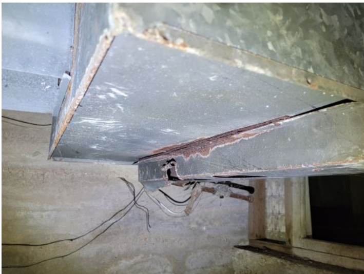
Rusted gas furnace
