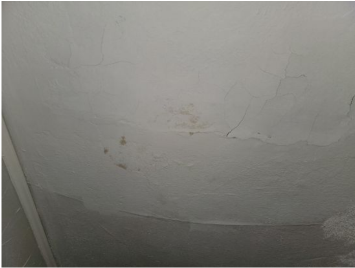
Sagging and damaged ceiling
