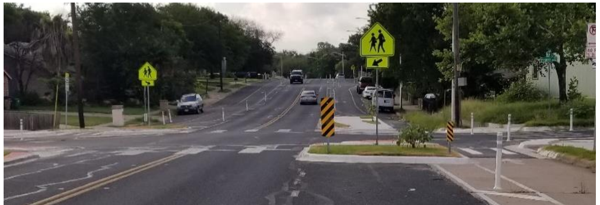
BEFORE AND AFTER PHOTOS OF TERI ROAD PROJECT WHERE EXISTING STREET SPACE WAS RECONFIGURED USING QUICK BUILD STRATEGIES (PAINT AND POST BIKEWAY PROTECTION), COUPLED WITH HIGHER QUALITY INTERSECTION IMPROVEMENTS.
