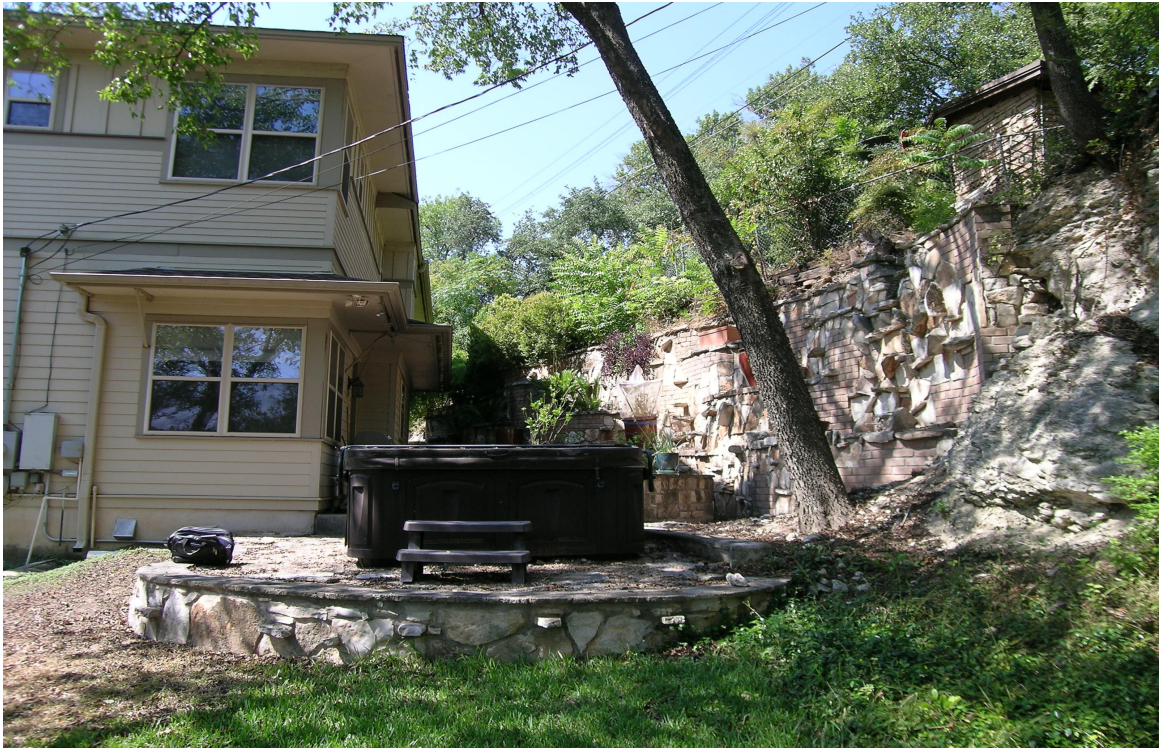
View of back of house with very tall retaining wall behind it. The retaining wall is about 25' tall per the survey.
