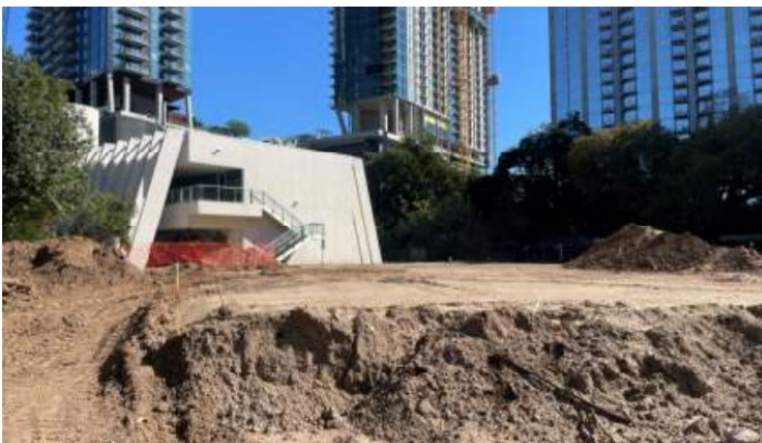
South Wing: Grading of building pad.
