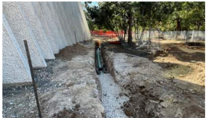
Zocalo: View of drainage installation
