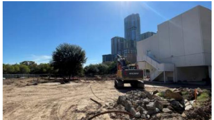
North Wing: Grading of building pad.
