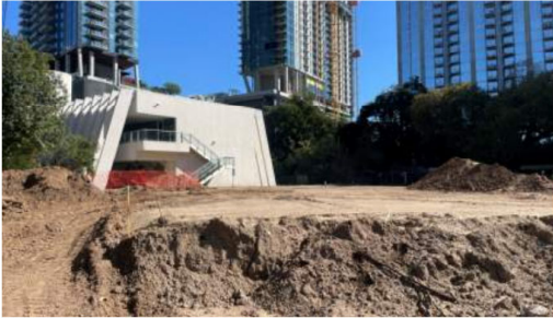
South Wing: Grading of building pad.
