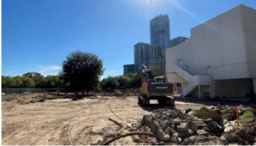
North Wing: Grading of building pad.
