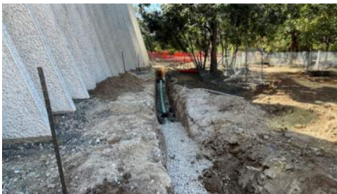
Zocalo: View of drainage installation
