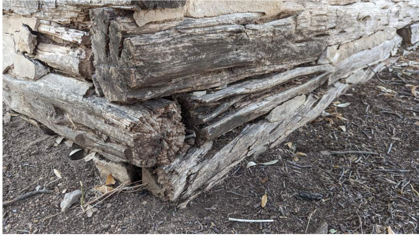
TYPICAL LOG, CHINKING, AND DAUBING CONDITION
