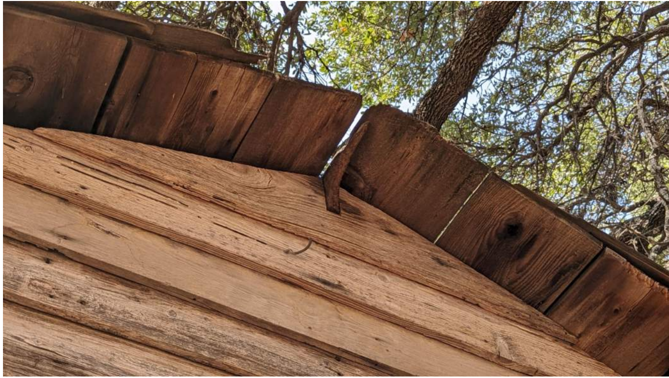
RIDGE BEAM, GABLE END LAP SIDING, ROOF SHEATHING AND CEDAR SHINGLES
