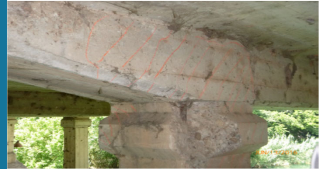
Delamination of Beams
