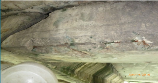
Spalling Concrete in Bridge Structure
