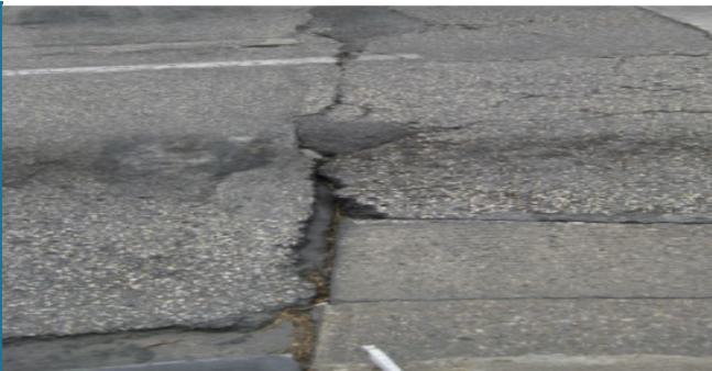
Cracking in Deck
